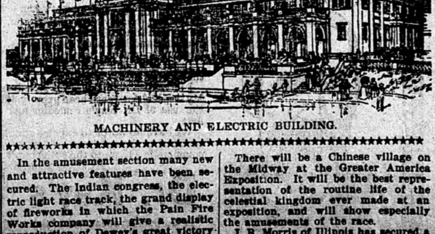
MACHINERY AND ELECTRIC BUILDING.
