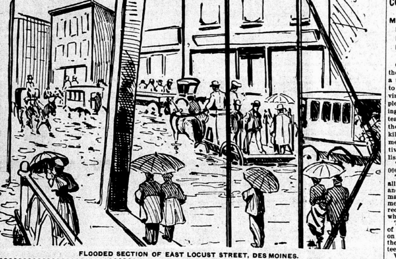
FLOODED SECTION OF EAST LOCUST STREET, DES MOINES.
