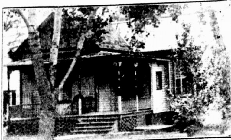
This is the home of Mr. and Mrs. Wm. Coalson 291 1/2 Center street, it is nine rooms entirely modern.
