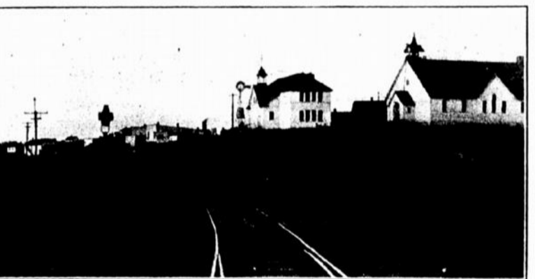
A View of East Buxton—A. M. E. Church and Private School Building.
