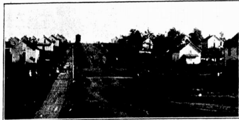
View of Main Street looking South.
