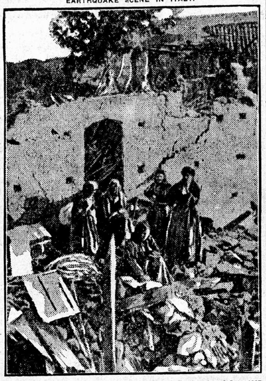
Calabrian Family Among Ruins of Their Home, Earthquake of Oct., 1907.
