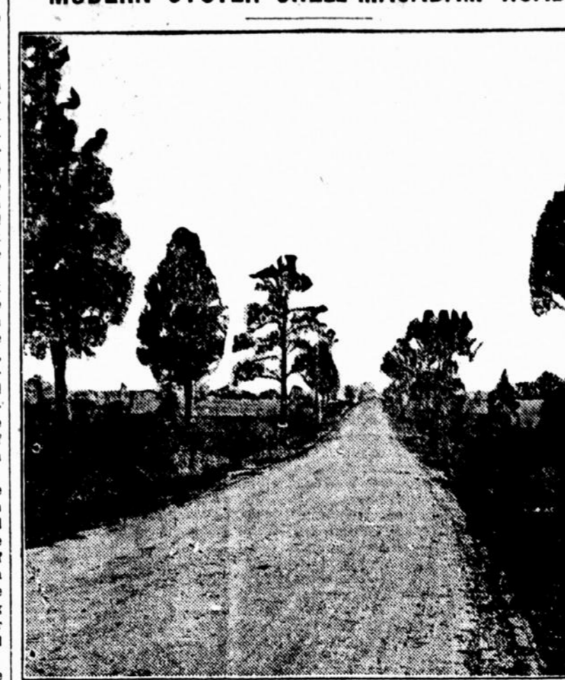
The illustration shows a modern Oyster Shell-Macadam Road Between East Newmarket and Mt. Holly in the State of Maryland.
