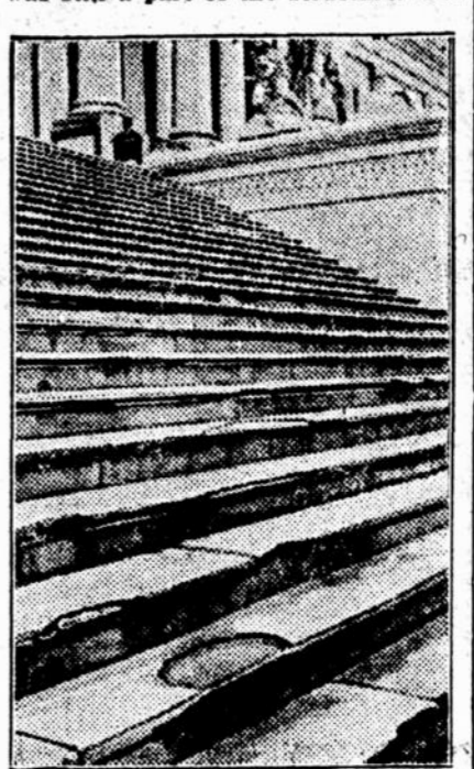
The Battered Steps at the East Entrance of the United States Capitol Which Are to Be Replaced After More Than Eighty Years' Service.
