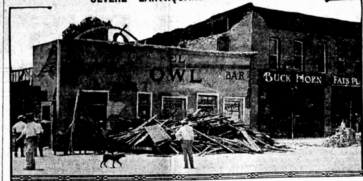
This photograph of a block of buildings in Mexcala gives some idea of the damage done by the recent earthquake that shook the Imperial valley in the southern part of California.
