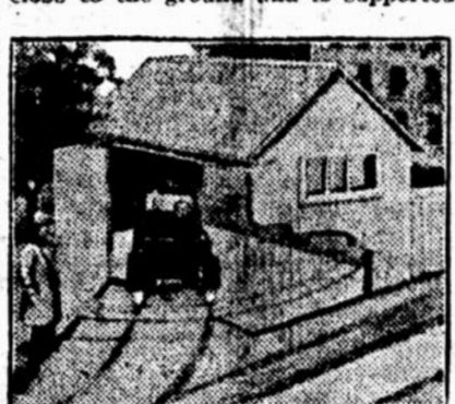
This Side Door, to Which a Low Platform Supported by Wheels Is Attached, Makes a Garage Facing on a Narrow Alley Easily Accessible.
