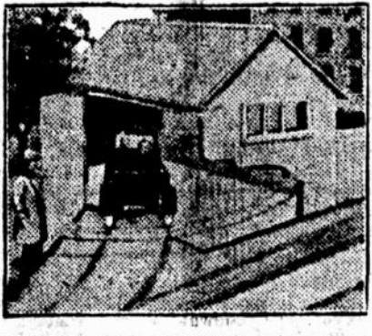
This Side Door, to Which a Low Platform Supported by Wheels is Attached, Makes a Garage Facing on a Narrow Alley Easily Accessible.
