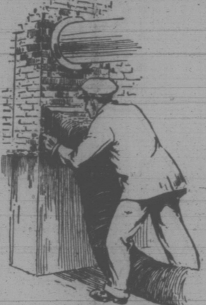
Removing Soot Accumulations From the Chimney is No Longer a Dirty, Messy Job. A Giant Vacuum Cleaner More Thoroughly Cleans the Chimney Than is Possible by Hand.
