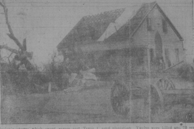
Cyclone storms which swept across east Texas struck with greatest force at the Arch Murry plantation near Grapeland. This photo shows the damage to crops and buildings. Twelve were killed and 70 seriously injured by the tornado which caused untold damage to crops and buildings.
