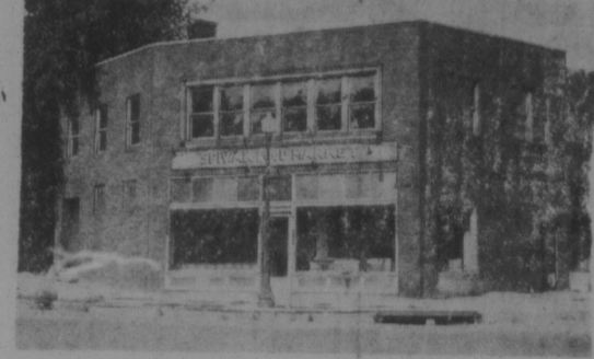
Building at 1333 Keosauqua way which will become USO service center.
