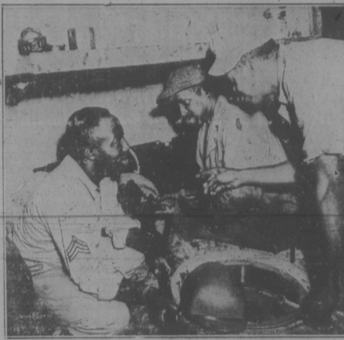
Released by U. S. War Department Bureau of Public Relations NEW GUINEA—Sergeant Robert B. Gibson of Chicago, Illinois, and Corporal Willie Lagree of Orlando, Florida, repair axle of one and one-half ton truck.
