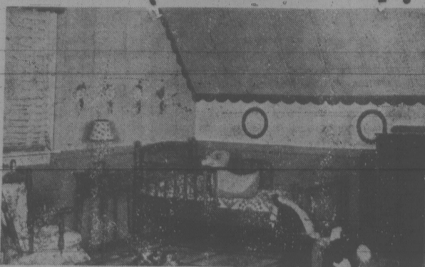
Wall board of several colors was used to turn unfinished attic into an attractive room for a child. Scalloped border was cut from the board.
