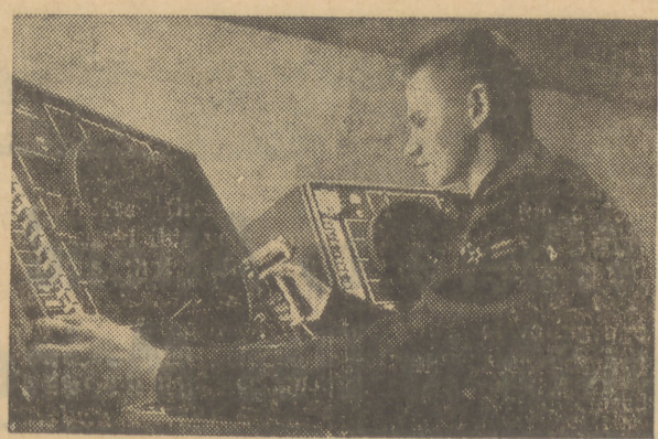
NEW IDEAS IN COMMUNICATIONS — Telephone circuits connect radar warning systems to the nation's defense watchposts. Above, at a SAGE Direction Center, an airman is using a photo-electric light gun to "question" an electronic brain on an approaching plane's identity. At left a young lady is holding a new "traveling wave tube," the key to a new transmission system that will more than double the communications capacity of trans-continental radio relay routes.
