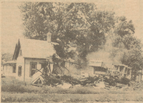
The house, half demolished, awaits the final blows from the bulldozer. The bulldozer sits almost in triumph
