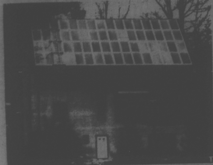
ROOFTOP SOLAR collector panels with inner glazing of "Teflon" Solar Film absorb the energy for this architect's house.
