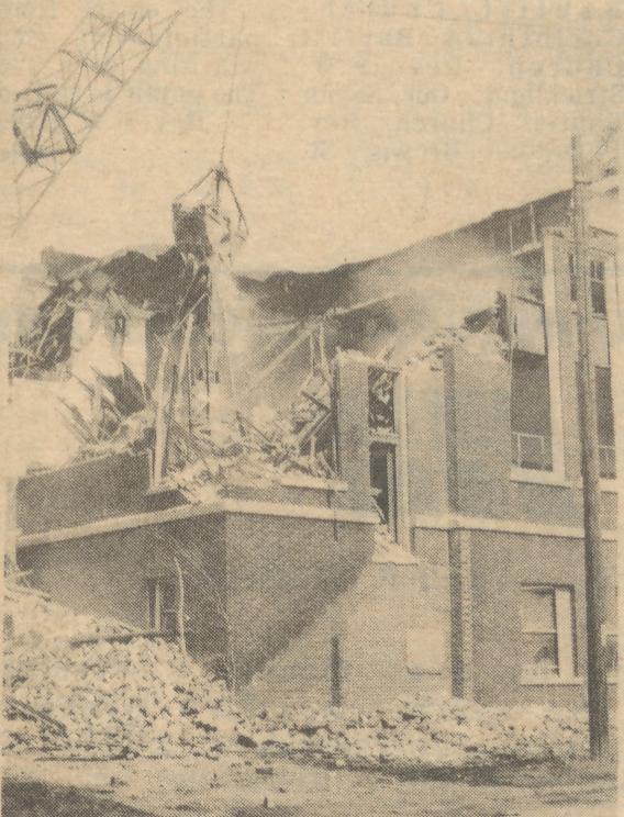
Old St. Paul church being demolished.
