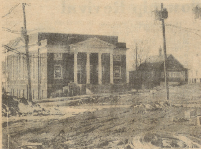
Old St. Paul structure, 12th and Crocker Sts., just prior to demolition,
