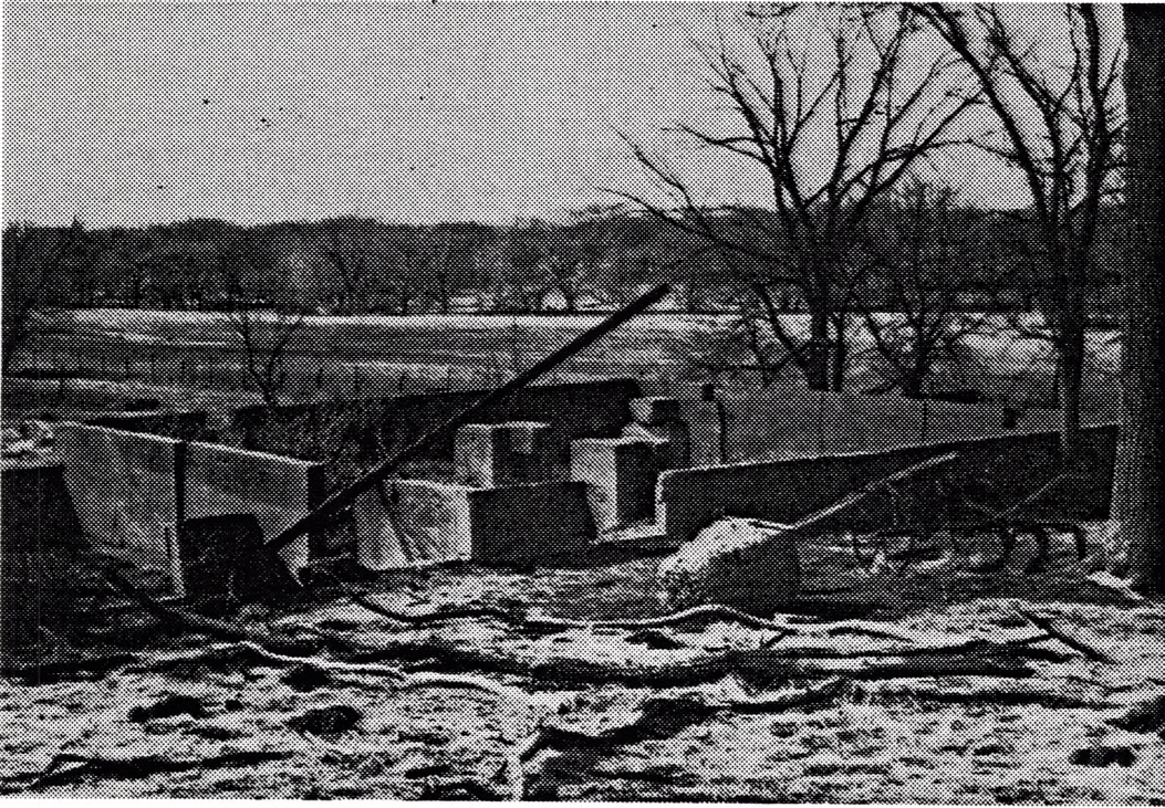
Figure 17. Foundation of White House Hotel, circa. 1960. Courtesy: State Museum and Archives.
