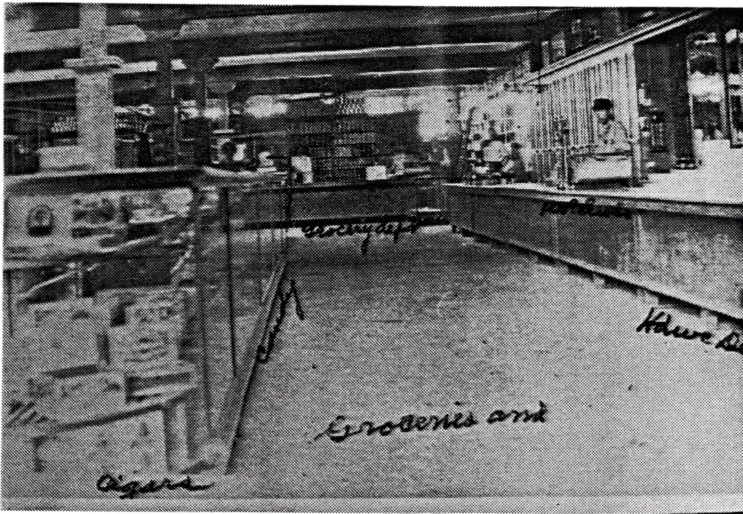
Figure 28. Interior of Company Store, Monro Mercantile Company. Courtesy: Dorothy Schwieder.
