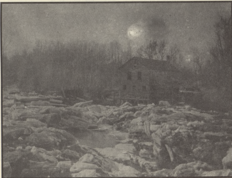
Old Mill on River at Lima. Abandoned about 1905.
