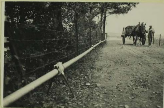
IRRIGATION PIPE Rubber joint Exp. Sta., Uni. of Bonn D104
