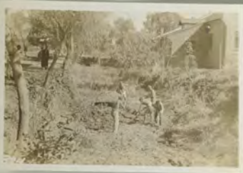
384. Removing soil from creek bed, NARB
