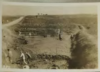
382. Removing soil from creek bed, NARB
