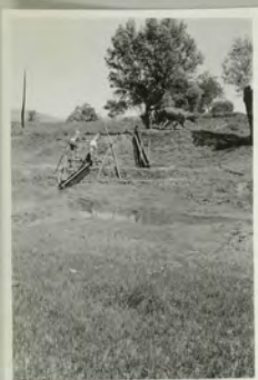
213. Water ladder, south of NARB
