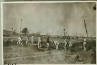
Grading at NAEC Shanghai
