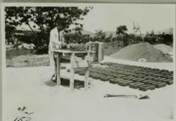
152. Making cinder concrete blocks for demonstration house
