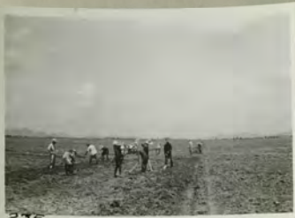
235. Making earth road by hand
