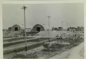
106. Quanset huts at NAEC Shanghai 4-26-47
