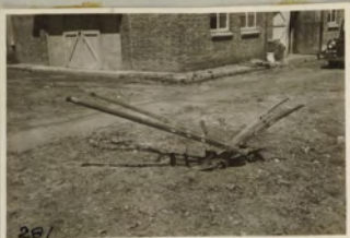
287 Chinese plow, Sub-station
