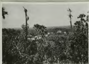
526 Farm buildings, Sheth farm
