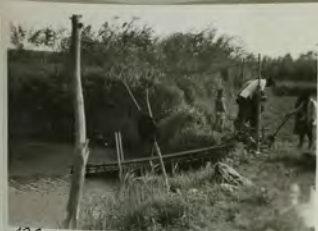
126. Water ladder, south of Nanking
