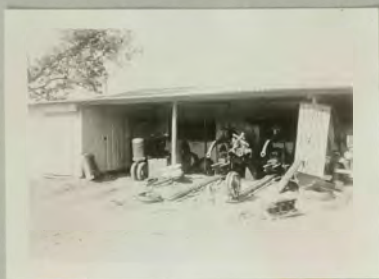
527 Repairing TD 14 & Farmall M Sheth farm
