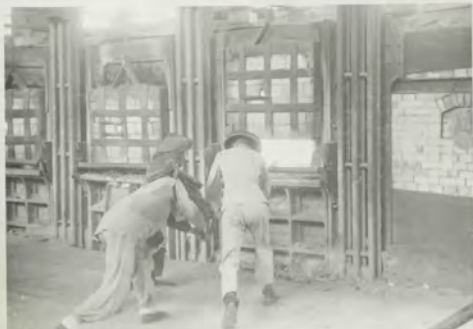
B4 Feeding steel billet into furnace
