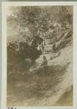
383. Removing soil from creek bed, NARB
