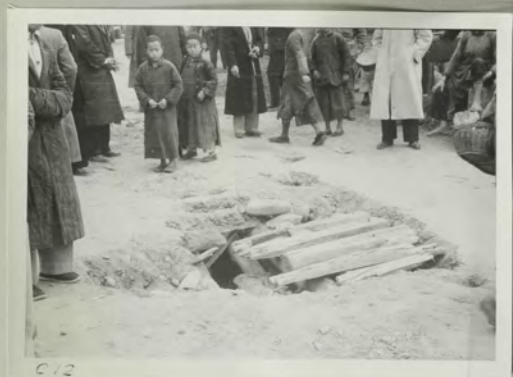
C12 Bridge needing repair
