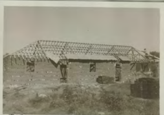
503 Earth wall construction on Uni. of Nanking Farm.
