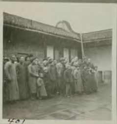
401. Group at Mu See Tow Lake, Reclamation Project at Community House, in rain, Feb. 1948
