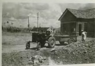
261 261. Farmall A & trailer, hauling road material
