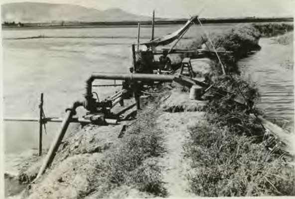
E. Pumping water with a five horse-power Diesel engine. This small plant has more than ten times the capacity of the plant shown in D.
