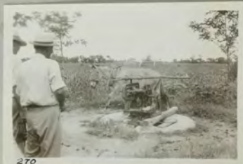
270. Pumping water with donkey
