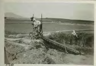
130. Water ladder - four men NARB 100 gpm - 3 ft. lift
