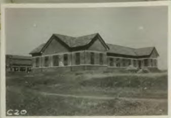
Agr'l. Eng. Building, NARB Feb. 1947
