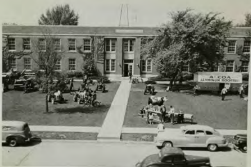
1948 Exhibit being assembled
