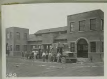
Arrival of first shipment of equipment NARB
