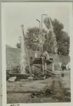
448. Tests of pumps, Farm machine factory, Taiyuan
