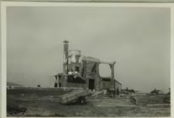
34. Ruins of former Administration Building, NARB
