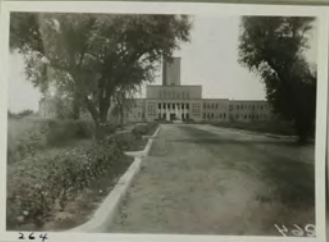
264. Main Building, NARB Substation Peiping
