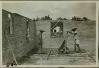
232. Pouring floor, demonstration farm house NARB
