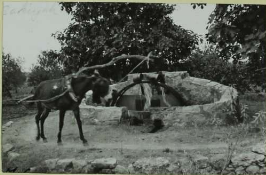
LIFTING WATER FOR IRRIGATION Near Valencia Spain
