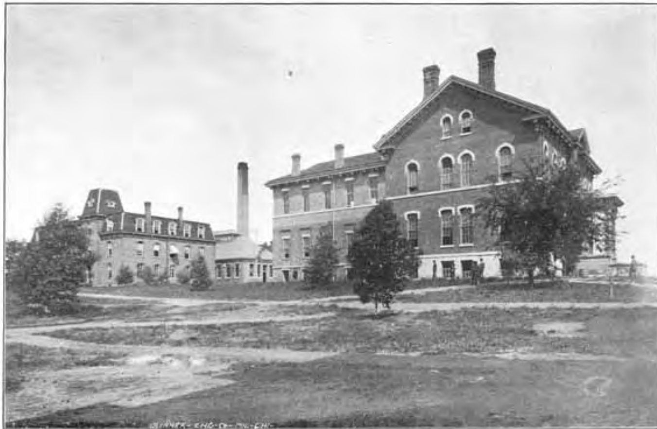
Engineering Hall. Physical and Chemical Hall.
