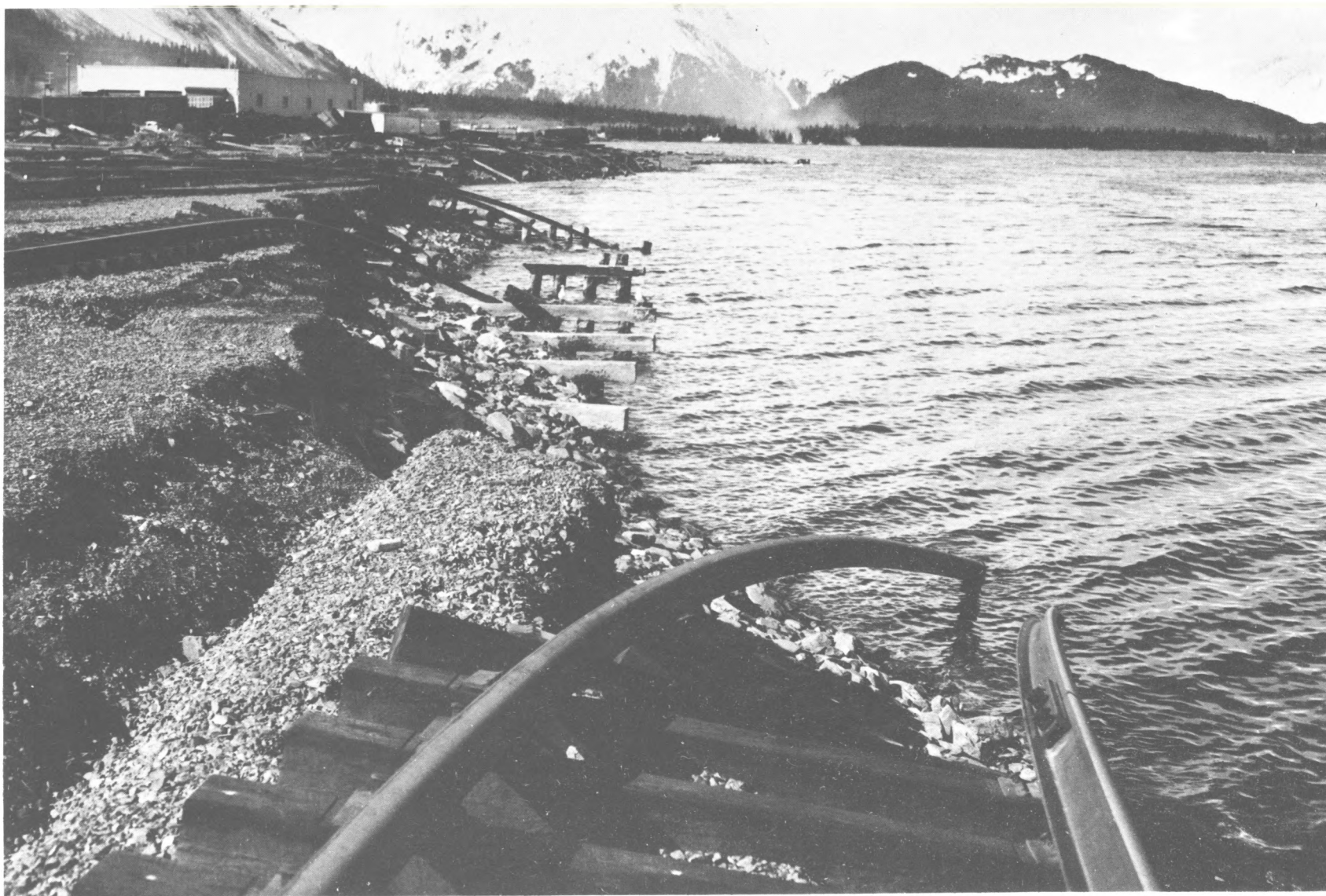
Seward, Alaska—The damaged Alaska railroad yard on the waterfront. A major portion of the waterfront slid into the sea as a result of submarine land slides.
