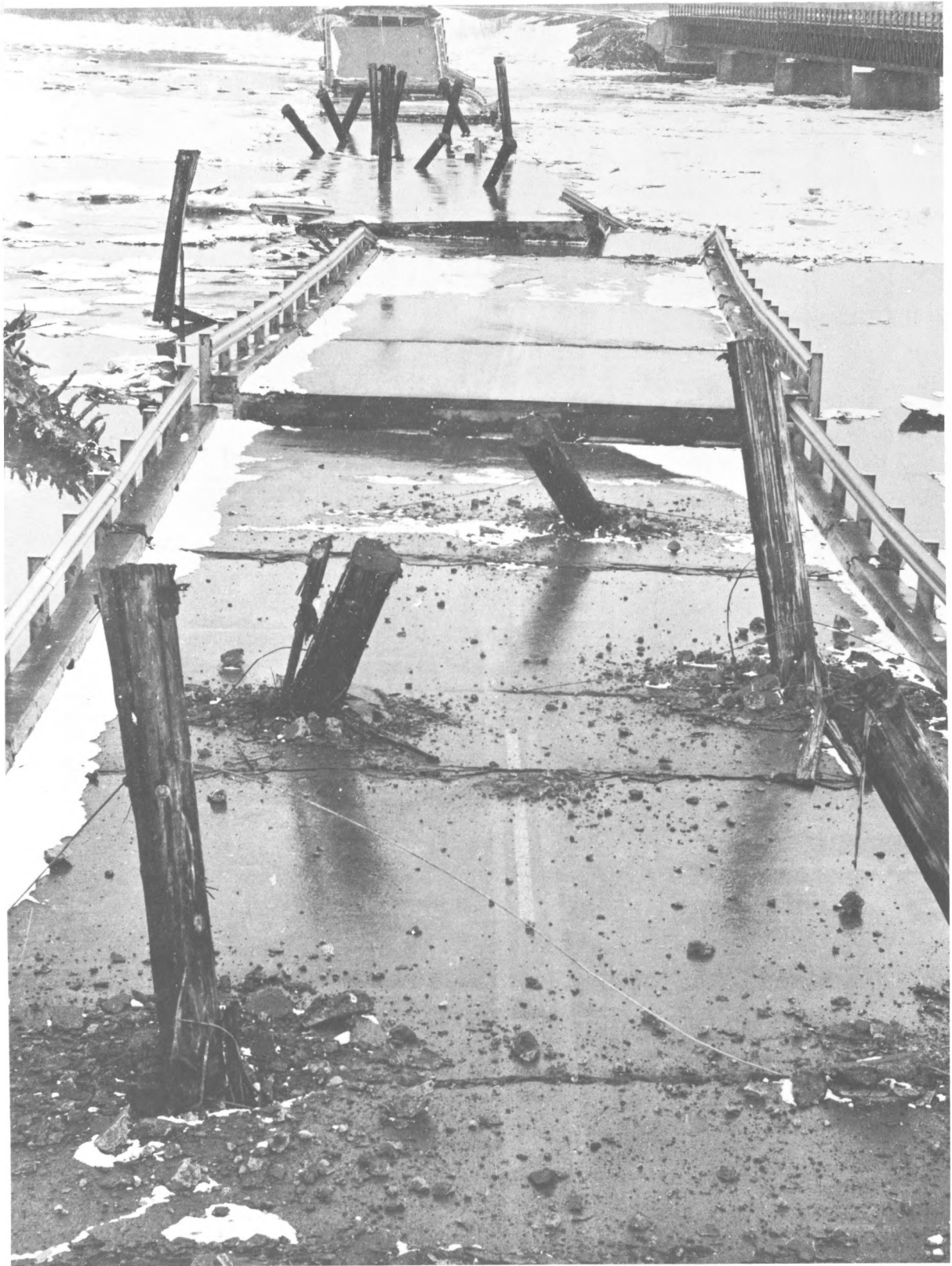
Portage, Alaska—One of the bridges which was wrecked by the earthquake.
