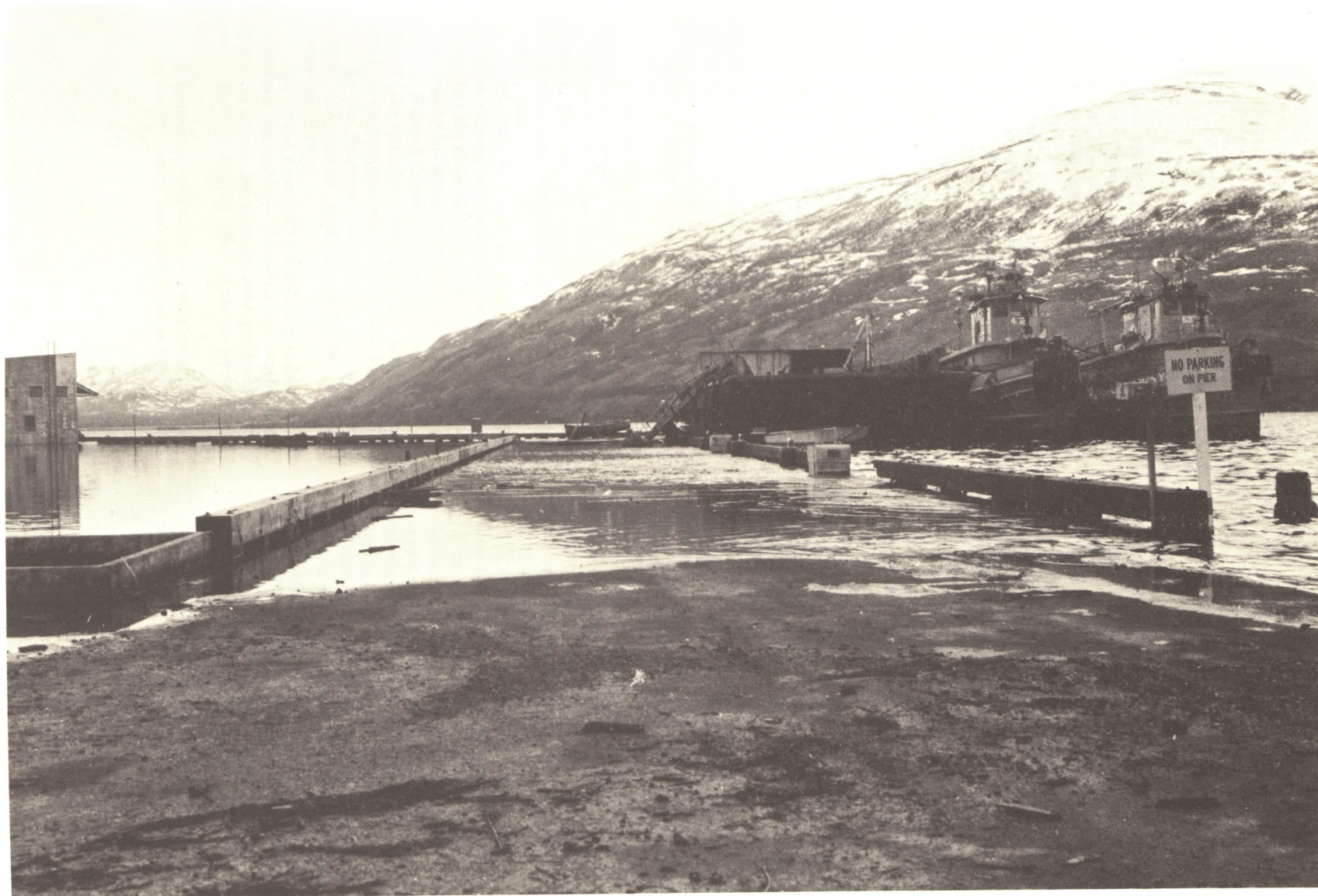
Kodiak, Alaska—The Kodiak marginal pier flooded by high tides after the land subsided following the earthquake.
