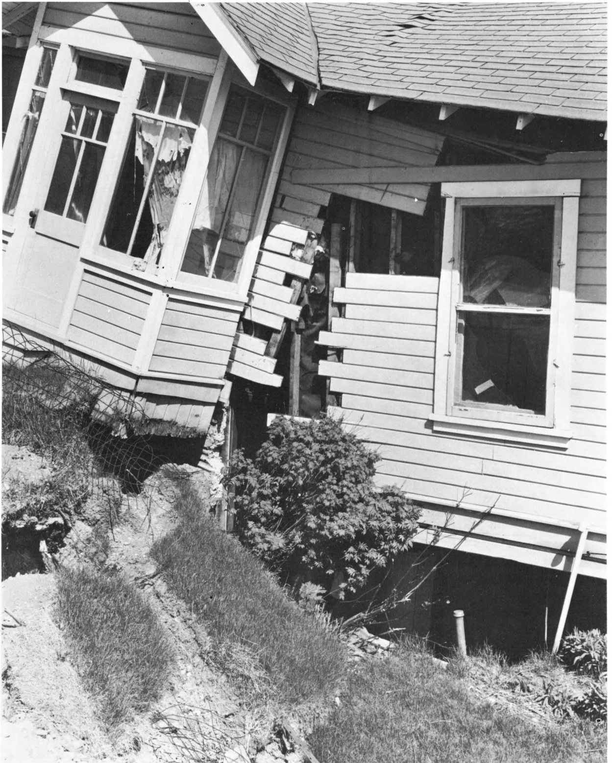
28.—Wrecked dwelling astride bounding fracture, L Street graben at Eighth Avenue and N Street. Damage caused entirely by ground displacement along fracture.
