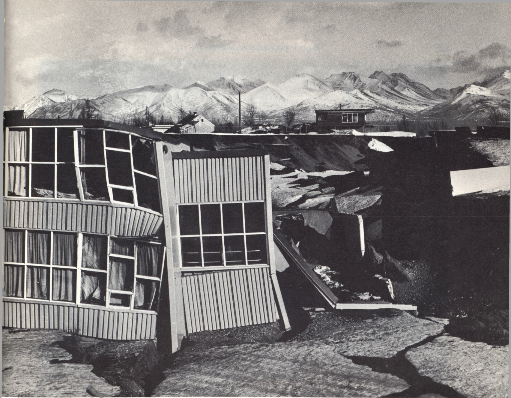
head of the slide. Net slip of the graben block is shown by the displacement of the roofline. Photograph by M. G. Bonilla.
