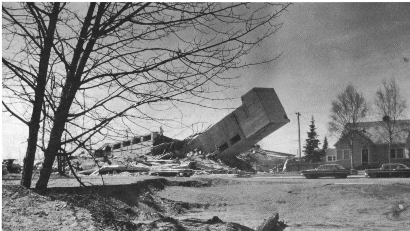
13.—Wreckage of six-story Four Seasons Apartment Building, Anchorage, Alaska. Canted elevator shaft at center. Large crack in foreground, filled in on M Street to restore traffic, passed beneath building.
