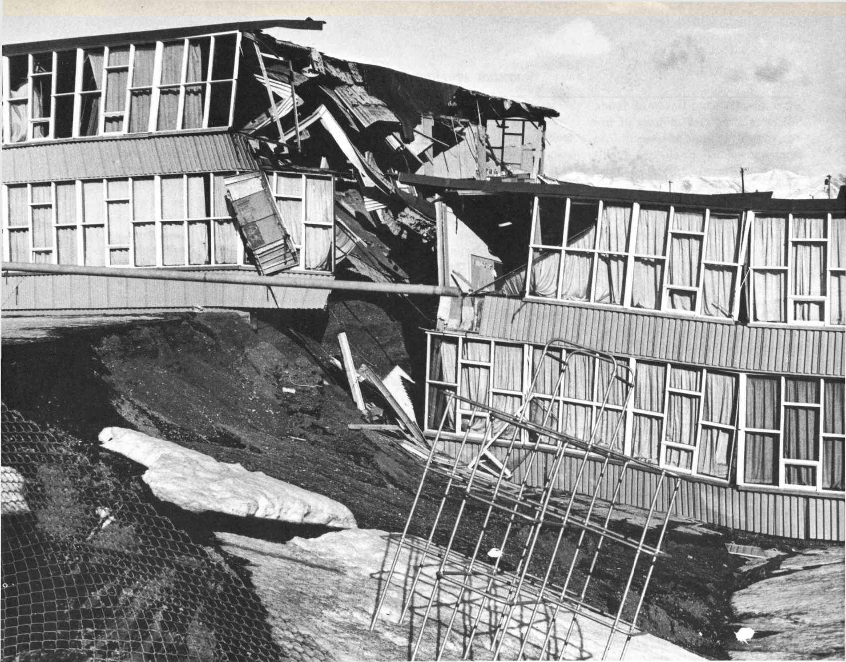
3.—Wreckage of Government Hill School. The south wing of the building, shown here, collapsed into a graben at the
