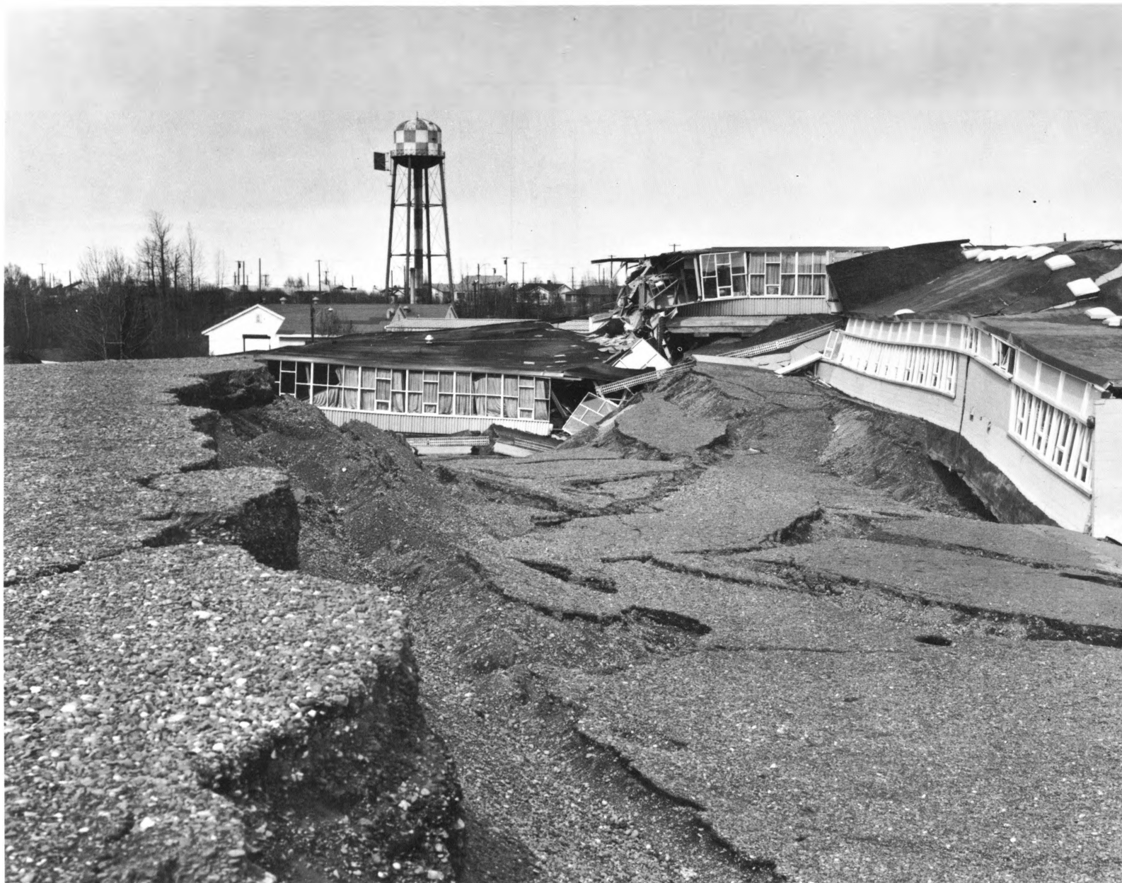
36.—Wreckage of Government Hill School as viewed from the playground, looking west. Graben in foreground is about 12 feet deep. Note undamaged water tower.
