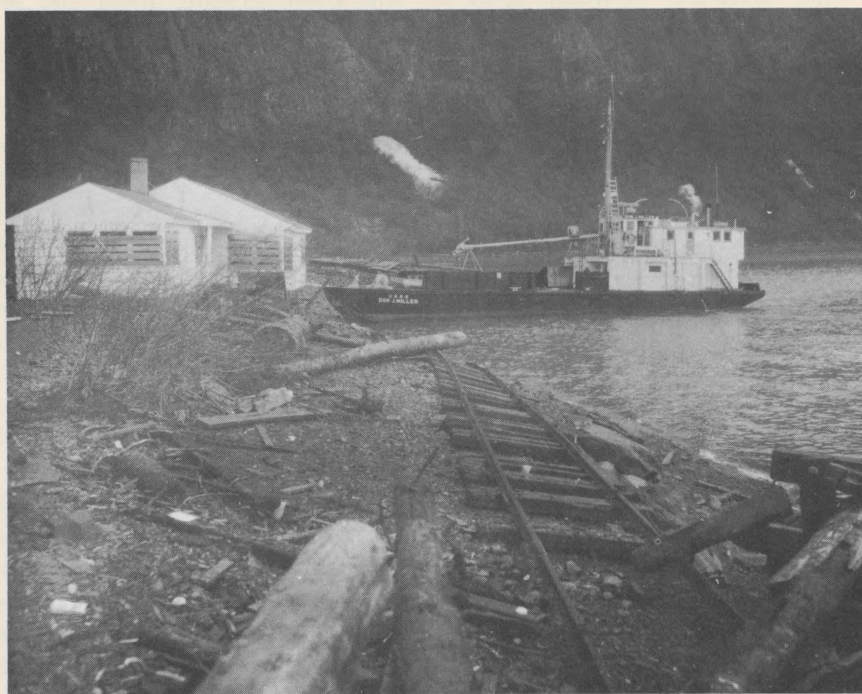
17.—View, looking north, of FAA station. Track destroyed by landslide. Bow of boat resting on scarp. Photograph by G. D. Hanna, 1964.
