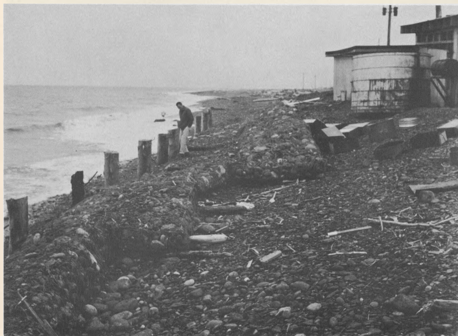
23.—Cobble-filled baskets placed on beach face to prevent erosion.
