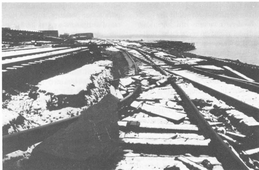
12.—Incipient landsliding along northern part of Seward waterfront. Fractured ground has subsided and rotated as landslide slump blocks.
