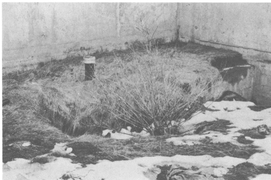
17.—Typical ground settlement resulting from the earthquake. Settlement is near the northeast corner of the powerhouse at the location of the septic tank.
