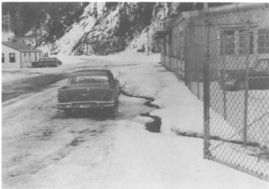
23.—Pavement damage caused by the earthquake. Cracks extend from the garage east along the north wall of the warehouse (right of photograph) and thence across the road to the project office (left of photograph).
