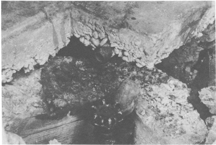
21.—Damage to the heating-system piping in the floor of the automotive repair shop caused by the earthquake.
