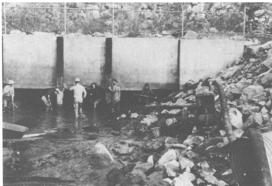
26.—Cleaning-up operation at the outlet of the tailrace conduit. Debris was deposited following the rupture of the tunnel intake at Eklutna Lake during the earthquake.
