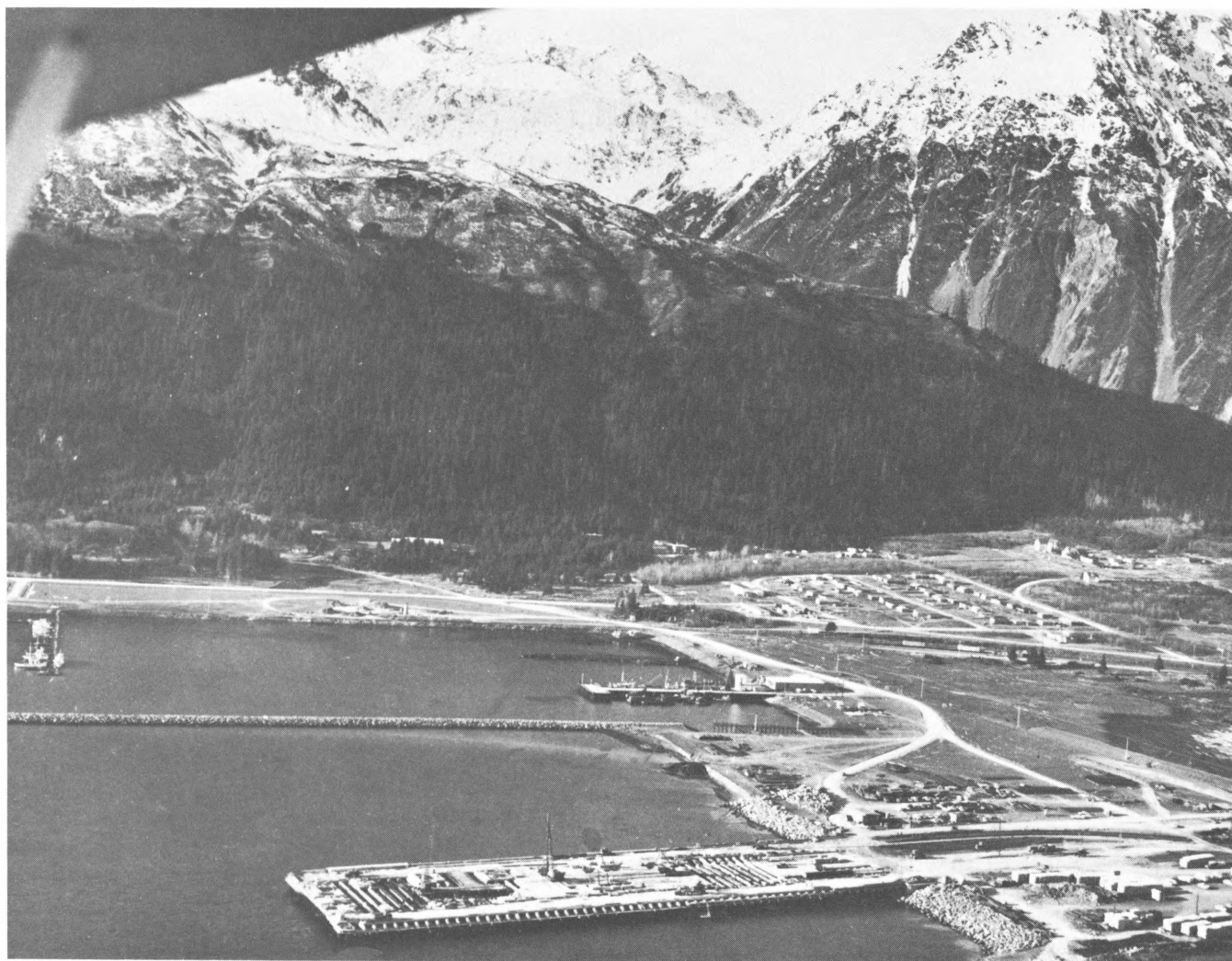
8.—Part of new small-boat basin and nearly completed railroad dock at Seward, November 1965. All former Seward waterfront facilities (to left of picture) were destroyed by submarine slides, waves, and fire. U.S. Army photograph.
