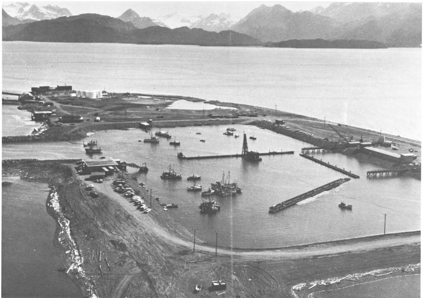
7.—New small-boat basin, excavated in end of Homer Spit. Former basin, on left side of the spit, was destroyed by a small offshore slide. The fact that the entire end of the spit is submerged by high tides because of tectonic subsidence and compaction necessitates dikes around new basin. U.S. Army photograph.
