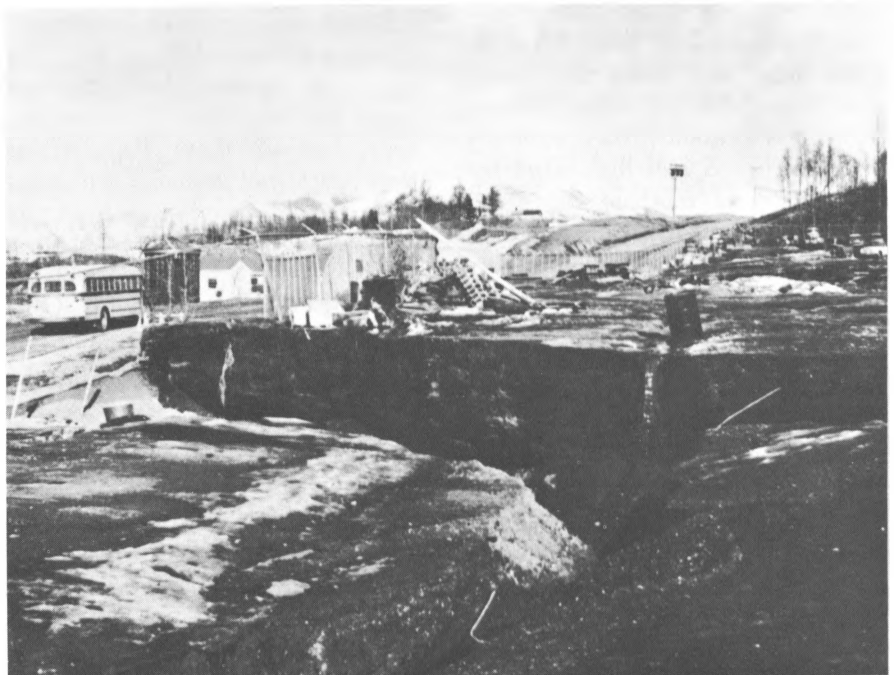
15.—Twelve-inch gas main, supplying fuel for municipal powerplant, was ruptured by landslide at Third Avenue and Post Road, Anchorage. Photograph by W. J. Stump.
