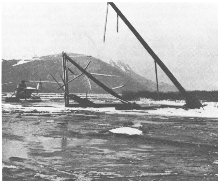
13.—Some power-transmission poles on Turnagain Arm were destroyed by liquefaction of silt foundation and by floating ice. Photograph by Chugach Electric Association, Inc.
