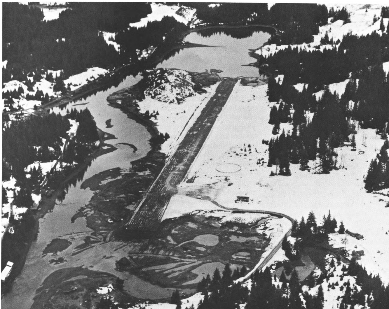
4.—Tectonic subsidence required raising of airstrip at Seldovia. U.S. Army photograph.
