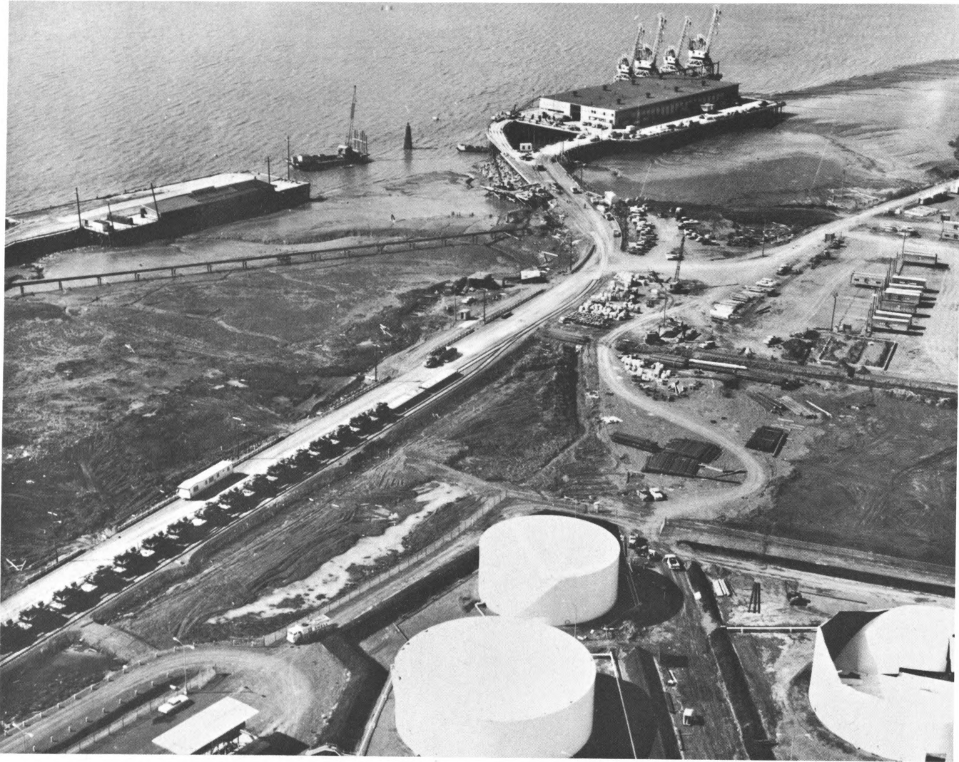
5.—Anchorage municipal wharf area shortly after the earthquake, at low tide. The main dock was only slightly damaged, but the older Army dock (upper left), was ruined. Vibration and ground fractures damaged some structures in the port area, including the petroleum tank (lower right). U.S. Army photograph.
