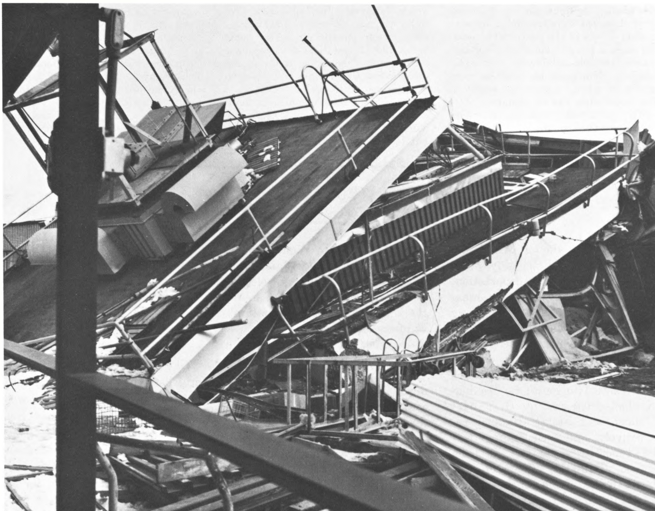
2.—Control tower at Anchorage International Airport, collapsed by earthquake shaking. Photograph by Federal Aviation Agency.
