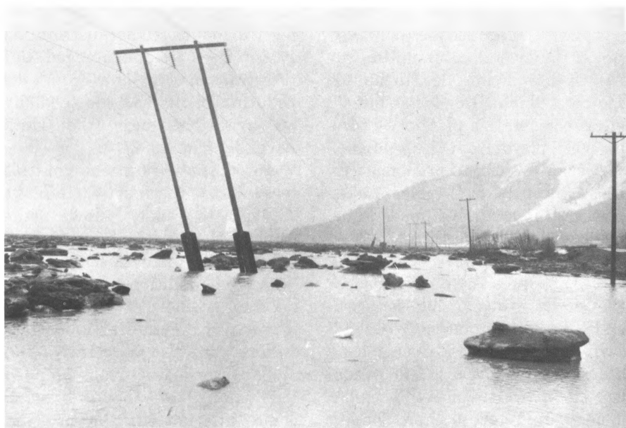
12.—Power and telephone poles along Turnagain Arm were tipped when the silt in which they were embedded was liquefied by earthquake vibrations. Photograph by Chugach Electric Association, Inc.
