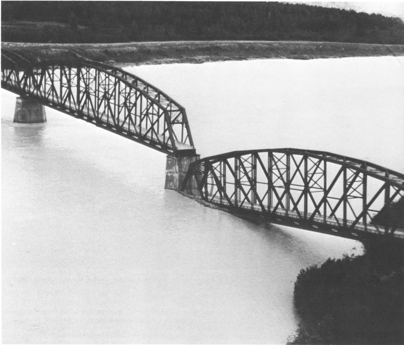
36.—Million Dollar Bridge, Copper River Highway ; No. 4 span off No. 4 pier. View is southwest.
