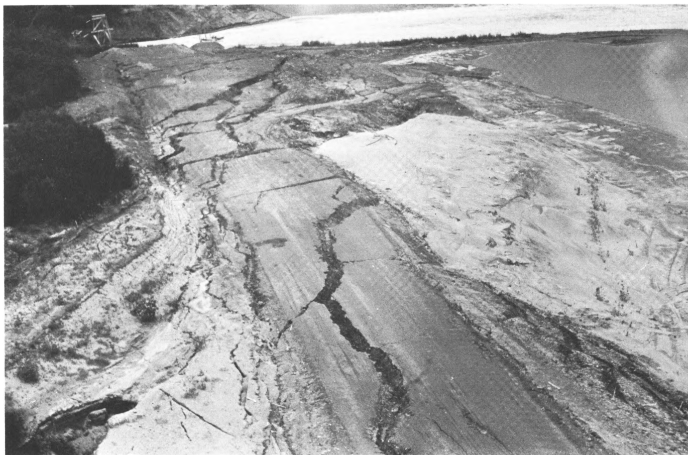
16.—Complex fractures with relatively large lateral and vertical displacements, produced by movement of saturated fine sand and silt toward free faces. View north near mile 58.5, Copper River Highway. The Allen River, which drains Allen Glacier, is in the background.
