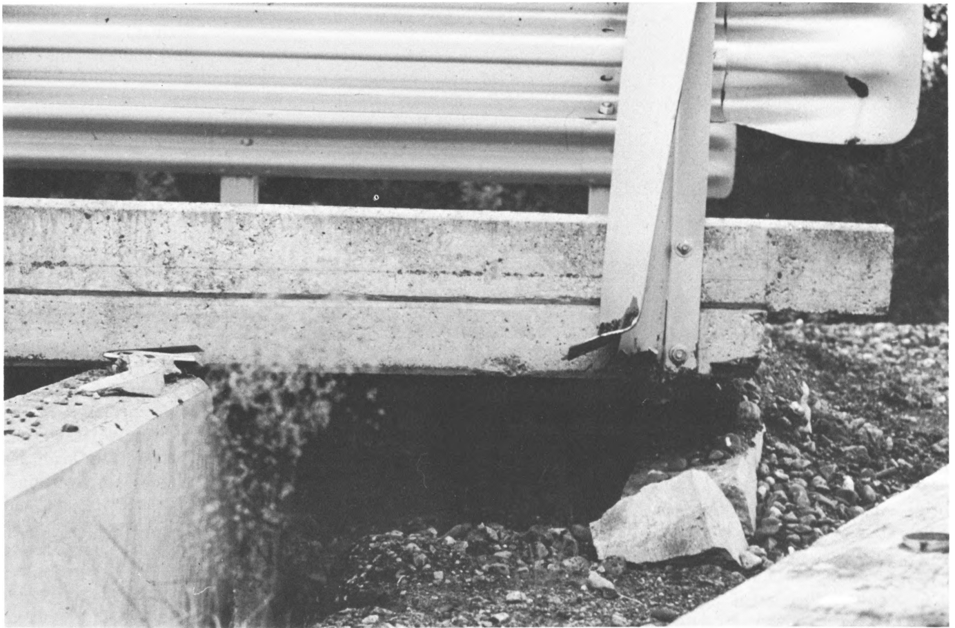
44.—North abutment of Clear Creek bridge 329, mile 41.0, Copper River Highway. Superstructure is displaced to the right relative to the abutment.
