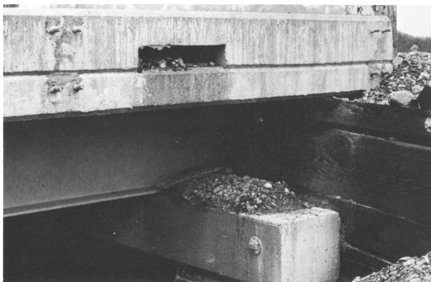
43.—East abutment of Scott Glacier Creek 5 bridge at mile 9.2, Copper River Highway. Superstructure is displaced about 2 feet to the right, relative to the abutment. Compare with figure 42.
