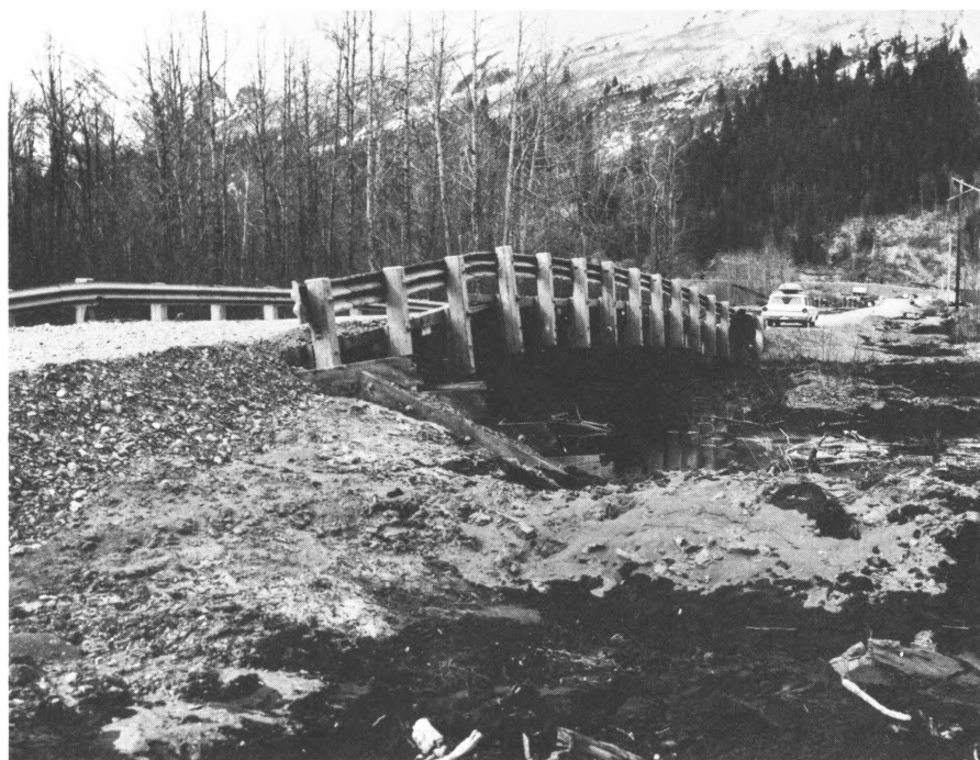
22.—View, looking west, of arched bridge at Snow River Crossing. Note that new fill in foreground was added to compensate for subsidence of approach fills and arching of bridge. Some of the original road fill had to be completely replaced. Photograph by D. S. McCulloch.
