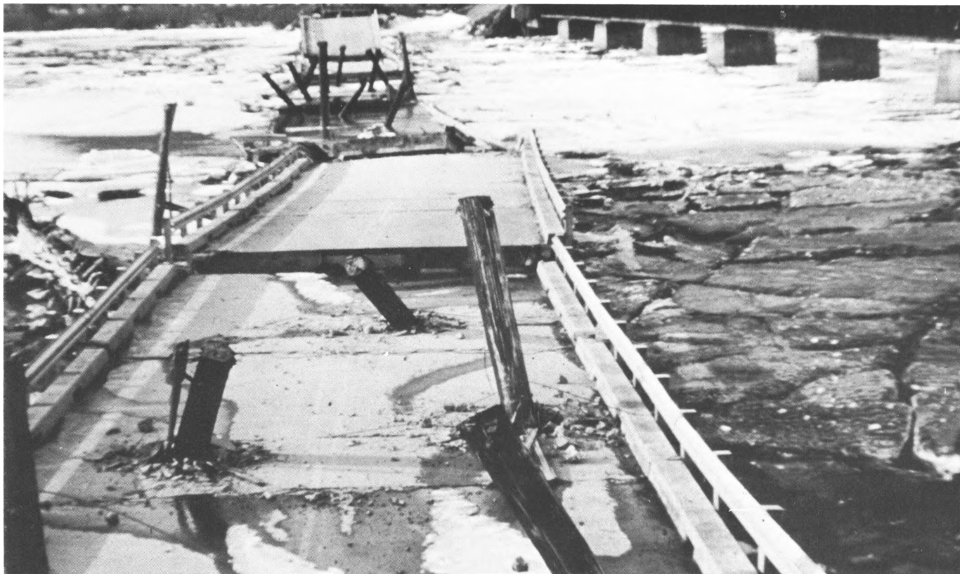
34.—Collapsed bridge across Twentymile River. Railroad bridge in upper right photograph did not collapse.
