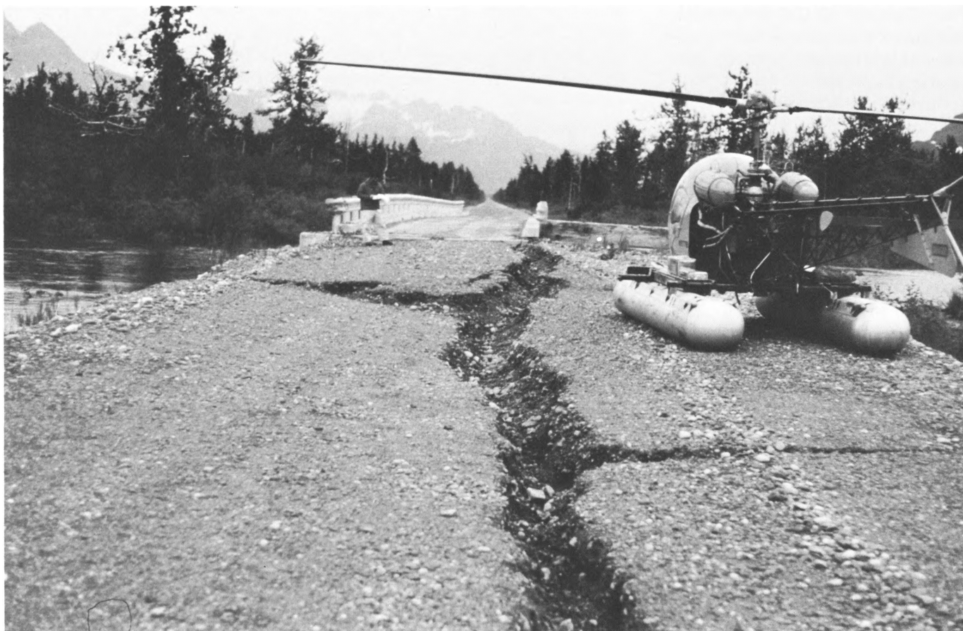
14.—Centerline fracture on unpaved Copper River Highway at south approach of Clear Creek bridge 329 at mile 41.0. Photograph by George Plafker.
