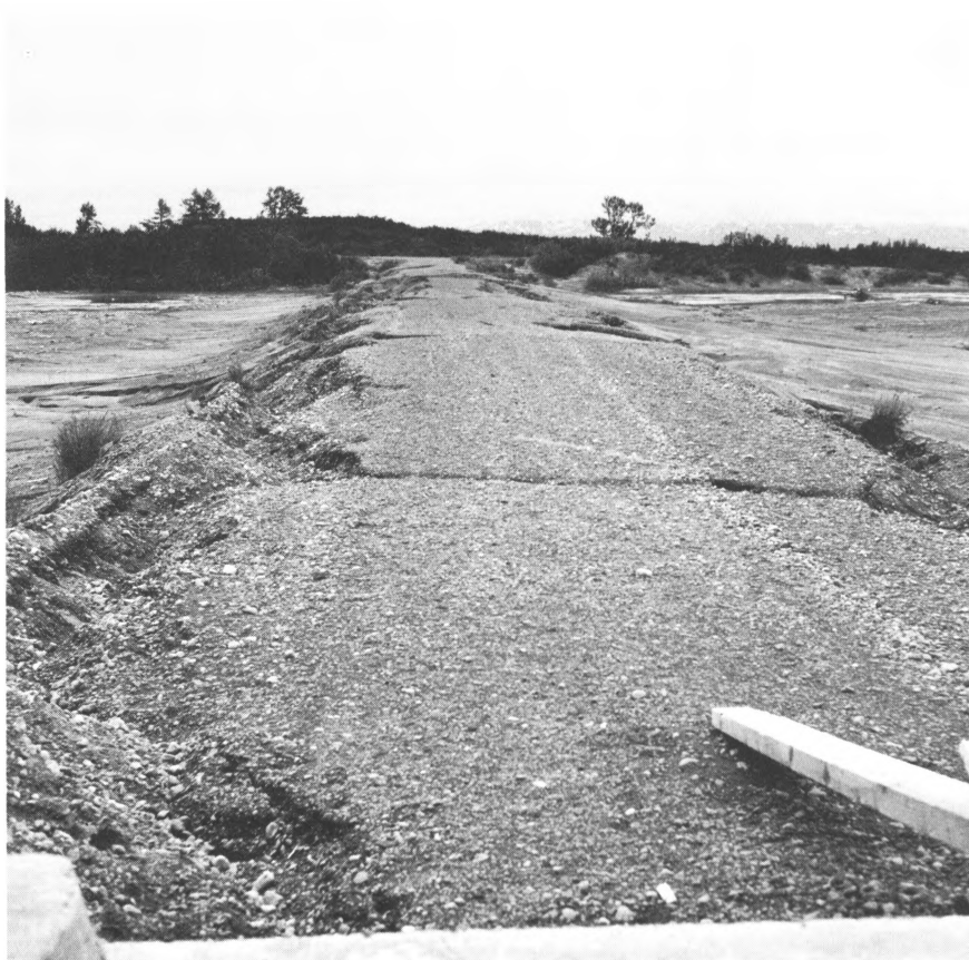
15.—Fractures normal to and along highway edge, Copper River Highway. Looking east from Copper River bridge 2, mile 27.1. Approach subsided 3 feet and fractured.
