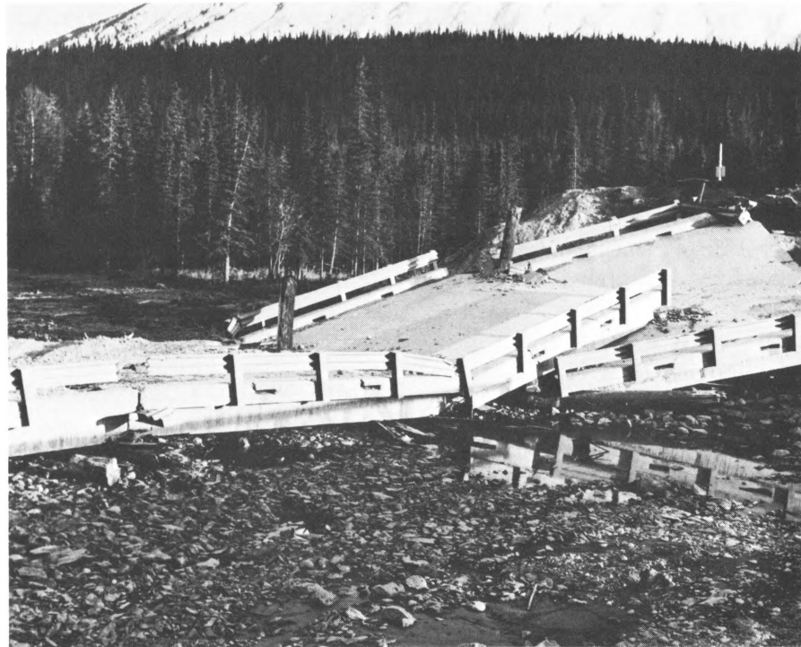
45.—Collapsed bridge across Kenai River at Kenai Lake, mile 48.9, Sterling Highway. Wood piles are driven through the collapsed reinforced concrete deck. Photograph by Helen Foster.
