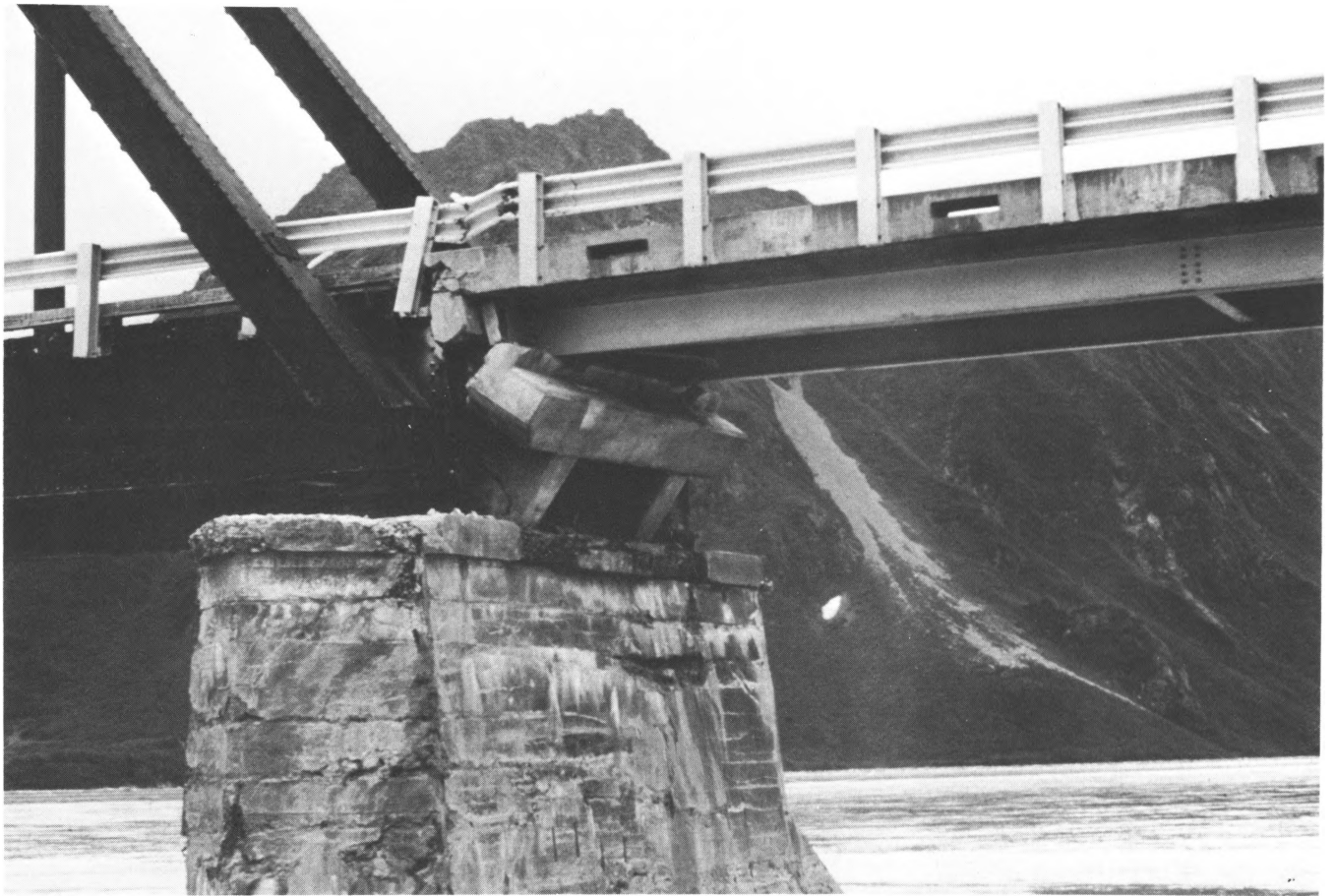
41.—Contact between steel truss and concrete deck on pier 26, Copper River 2 bridge, mile 27.1, Copper River Highway.
