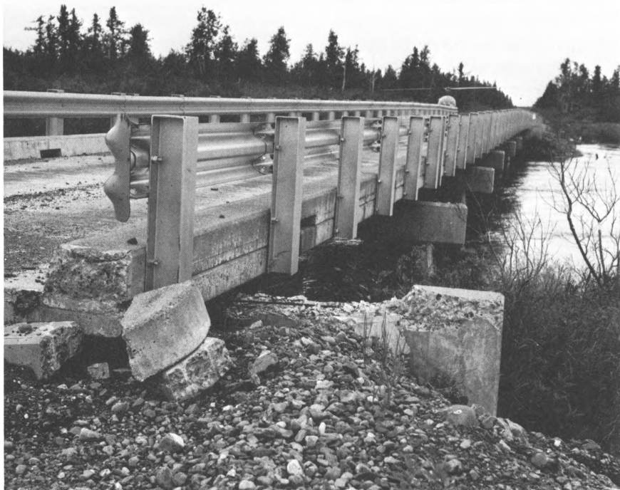
48.—North abutment of Copper River 9 bridge, 338, mile 36.1, Copper River Highway, showing displacement of deck laterally to the left relative to substructure. Photograph by George Plafker.
