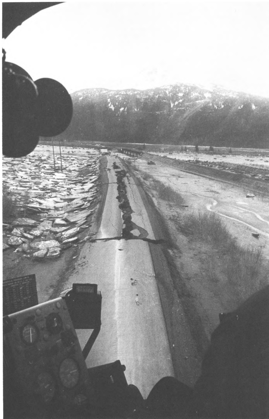
13.—View northwest showing conspicuous centerline fracture and more typical perpendicular fractures on Seward-Anchorage Highway between Portage and Twentymile River. Photograph by D. S. McCulloch.
