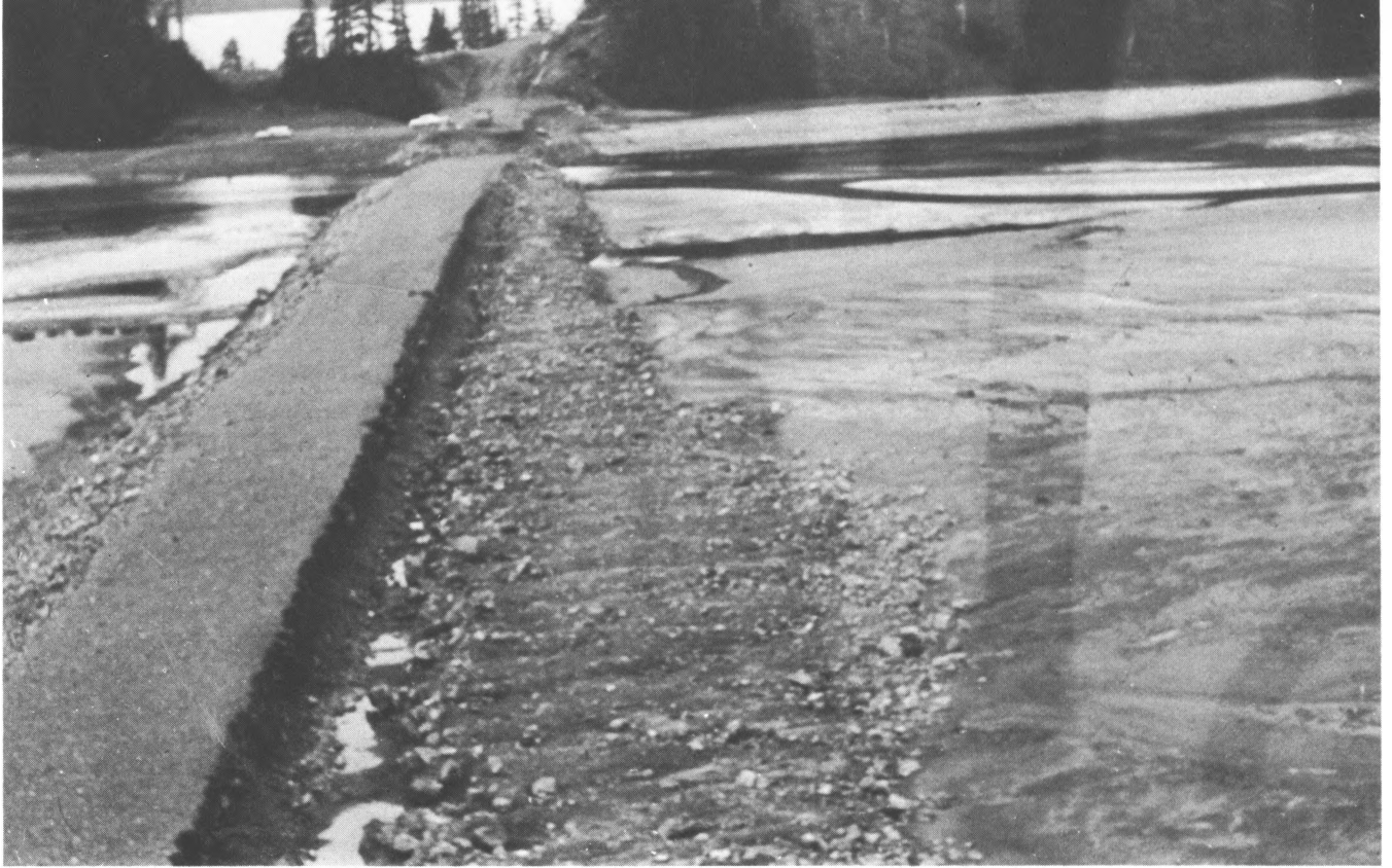
26.—Right side of Point Whitshed Road destroyed by seismic sea waves. Waves advanced over roadway from the left and cut sharp edge on right side of roadway. View northeast; Hartney Bay is to the right.
