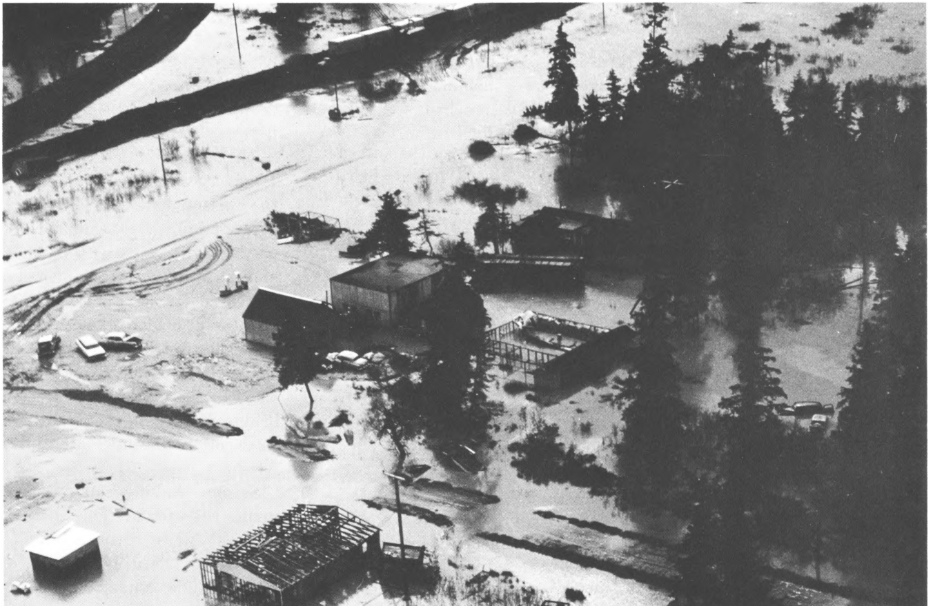
27.—View of Portage on Seward-Anchorage Highway during 28-foot tide, after regional subsidence caused by the earthquake. Highway is under water, just below railroad grade in far background. Photograph taken August 10, 1964.
