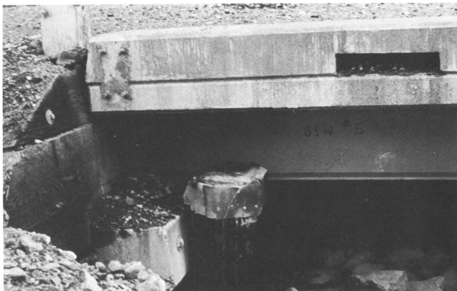
42.—West abutment of Scott Glacier 5 bridge, mile 9.2, Copper River Highway. Concrete cap displaced 2 inches to the left off the pile bent. Compare with figure 43.
