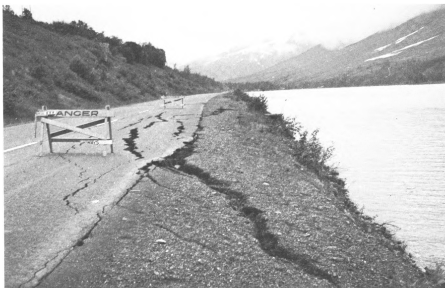
24.—Small landslide on Seward-Anchorage Highway near mile 44.5, along shore of Summit Lake.
