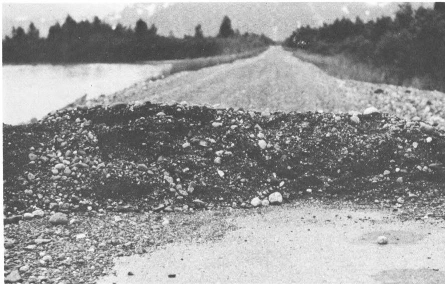
32.—Mound formed by bulldozing of approach fill against bridge deck (foreground), at north end of Copper River 12 bridge, mile 36.9, Copper River Highway.
