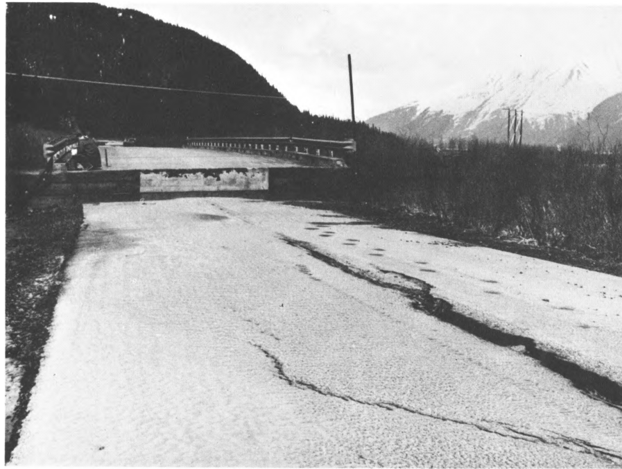
30.—Subsidence of bridge approach fill at Tidewater Slough 2 bridge, mile 76.4, Seward-Anchorage Highway. View is west. Photograph by Helen Foster.
