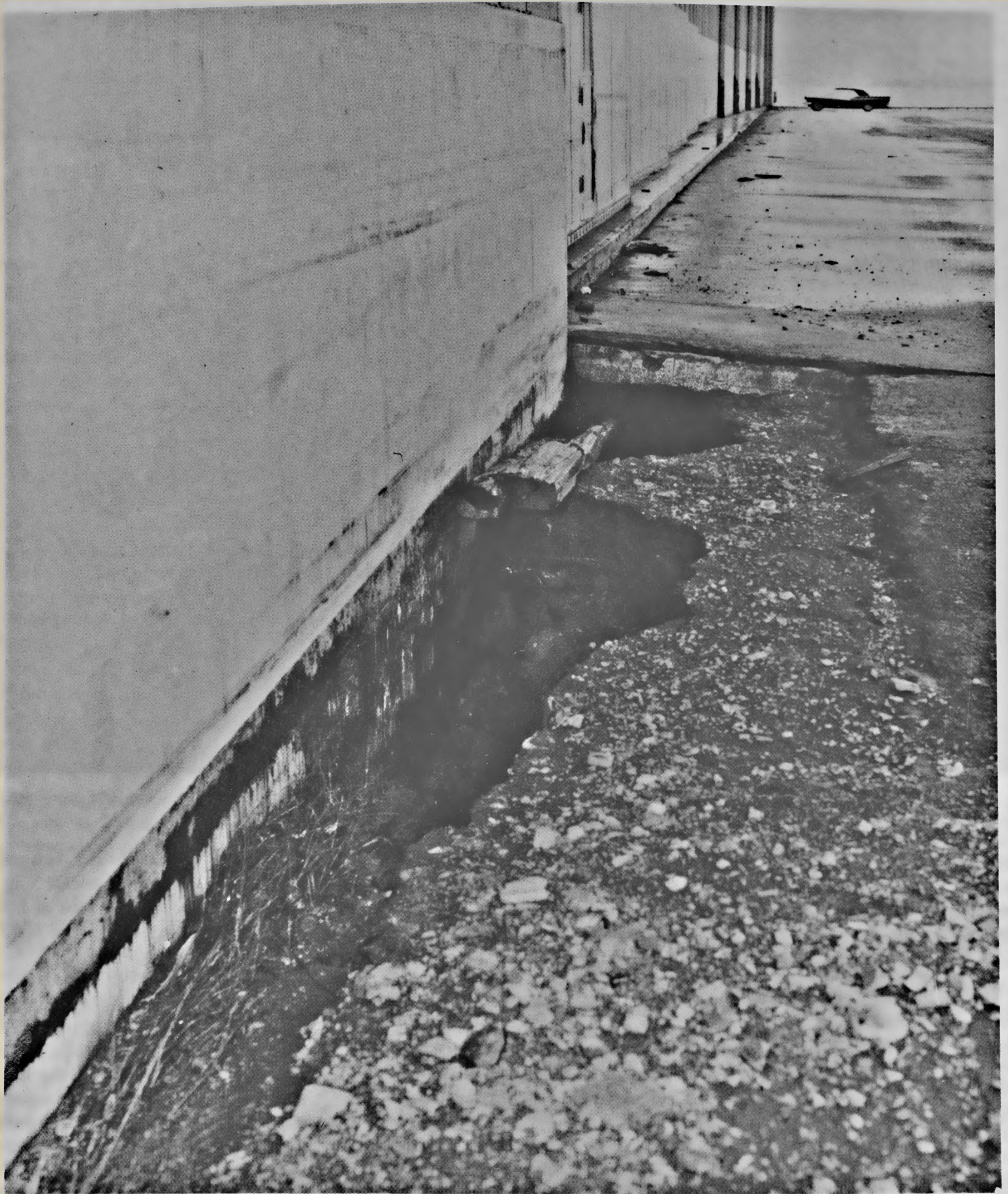
5.—Result of compaction of fill debris underlying asphalt aircraft ramp outside hangar at Kodiak Naval Station. Note the settlement of back-fill material adjacent to foundation of structure in the foreground. Photograph by U.S. Navy, March 29, 1964.
