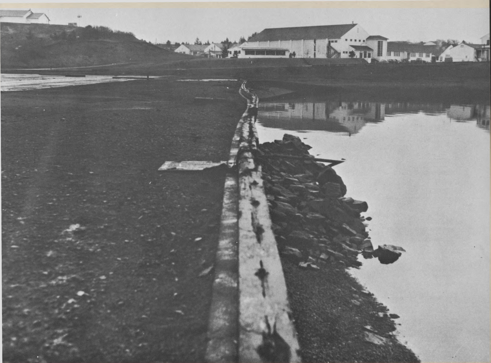
4.—Displacement of seawall toward Womens Bay, Kodiak Naval Station. View is east. Photograph by U.S. Navy, April 1, 1964.
