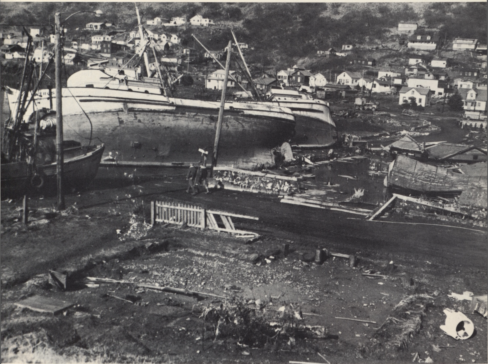
18.—Foundations of structures swept away by seismic sea waves, downtown Kodiak. View is west from intersection of Marine Way and Mill Bay Road. Foundation across Mill Bay Road was the Elks Bowling Alley; the boats are the Cindy , Albatross , and Hekla . Photograph by U.S. Navy, March 28, 1964.
