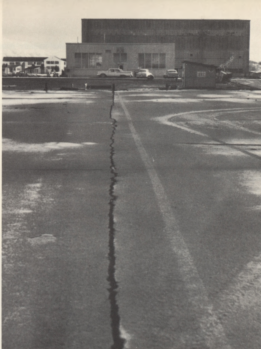
3.—East-west-trending fissure in aircraft parking ramp at Kodiak Naval Station. View is west. Photograph by U.S. Navy, March 29, 1964.
