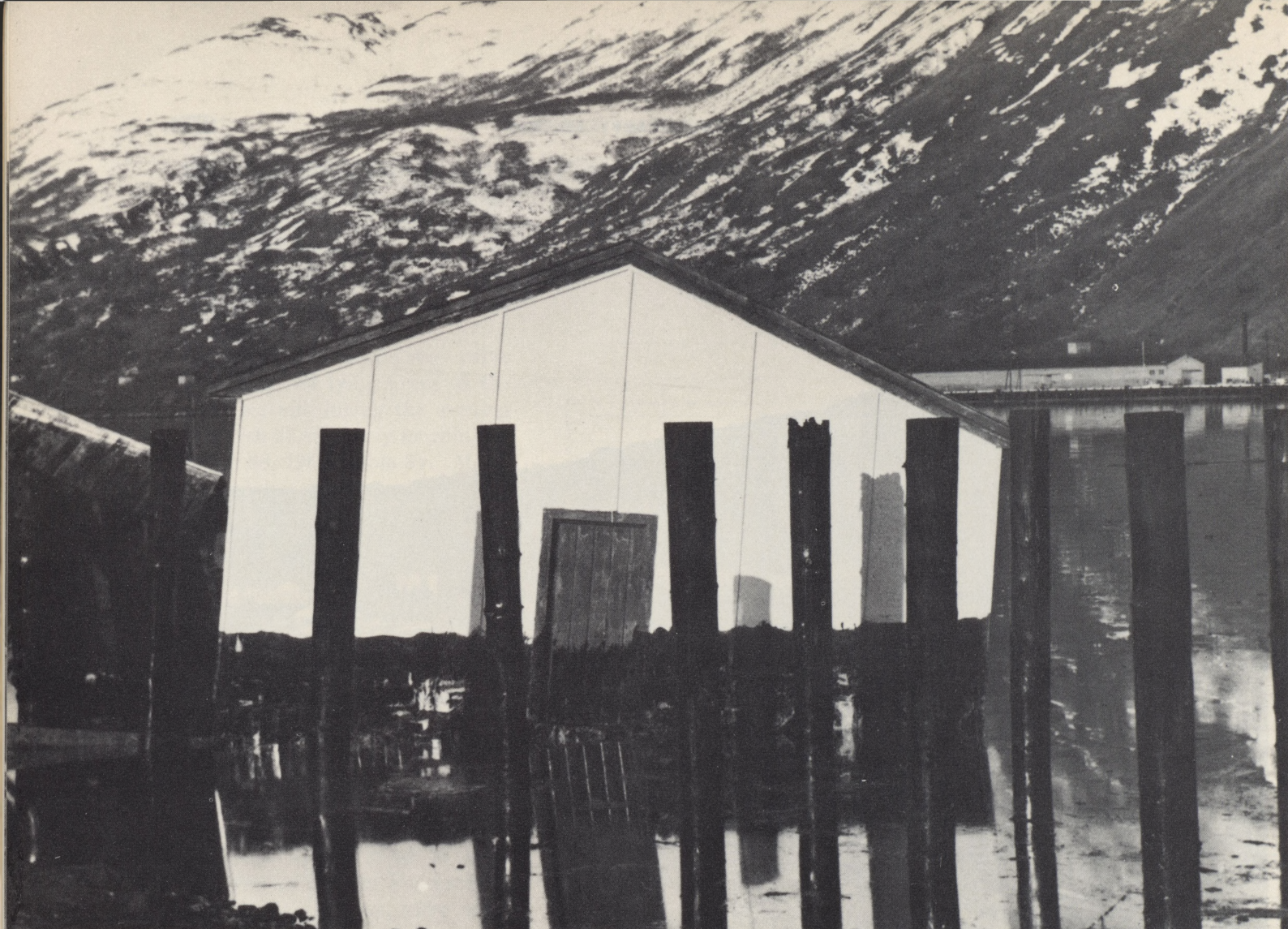
11.—Hobby shop swept off its piling foundation by seismic sea waves, Kodiak Naval Station. Black poles are piles upon which structure rested prior to the earthquake. Photograph by U.S. Navy, March 28, 1964.
