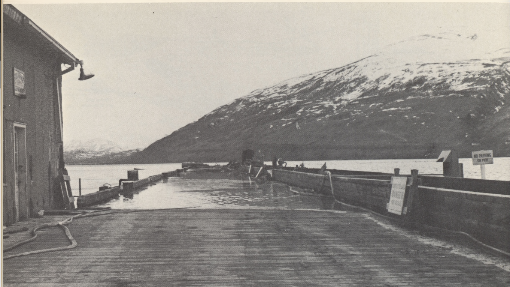
7.—Inundation of fuel pier during high tide at Kodiak Naval Station. Photograph by U.S. Navy, 12:59 p.m., April 12, 1964.
