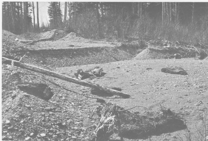
31.—High scarp ( 4\frac{1}{2} ft) of a rotational slump on the south side of Victory Creek on Lakeview delta.
