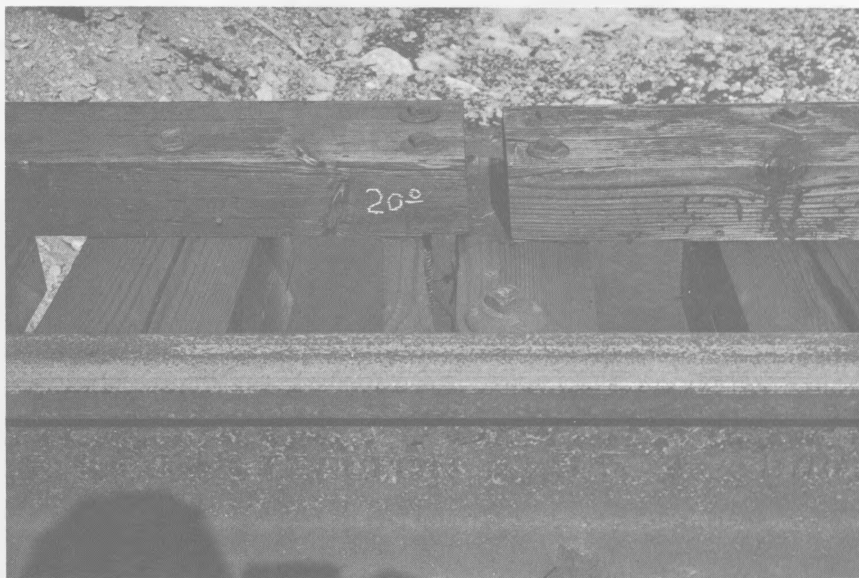
27.—Tension on Lakeview delta railroad bridge pulled guard timbers apart and split a tie.
