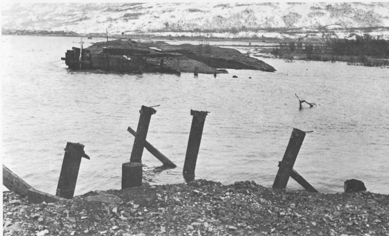
24. — Deck of highway bridge at Womens Bay washed away by seismic sea waves. Photograph by U.S. Navy, March 30, 1964.
