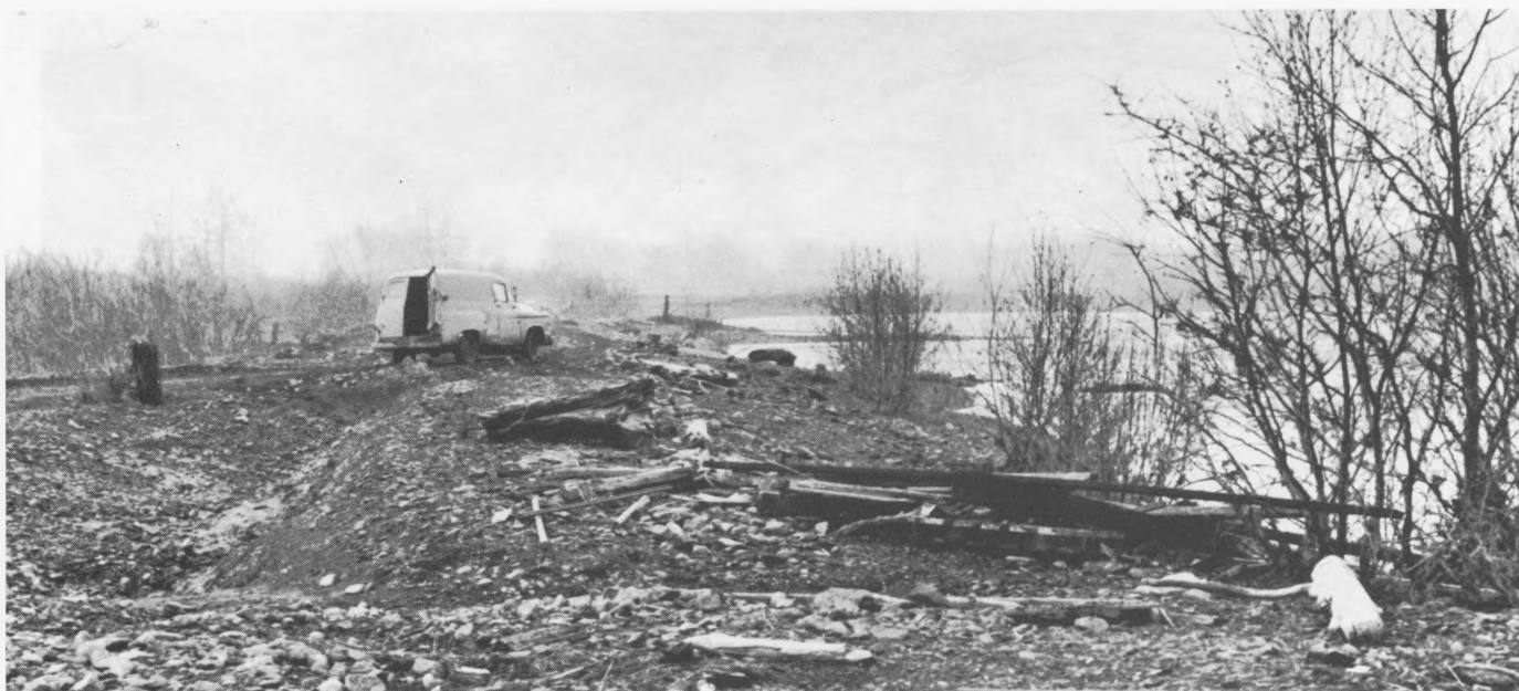
25. — Section of roadway along Chiniak highway at Womens Bay destroyed by seismic sea waves. Photograph by U.S. Navy, March 30, 1964.
