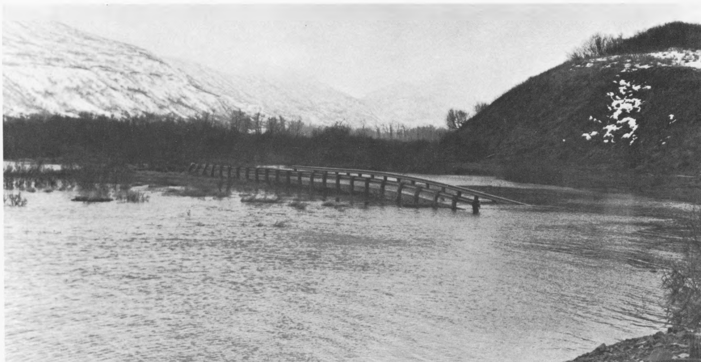
23. — Bridge at Womens Bay destroyed by seismic sea waves. Deck of bridge collapsed owing to destruction of piles. Compare with fig. 24. Photograph by U.S. Navy, March 30, 1964.
