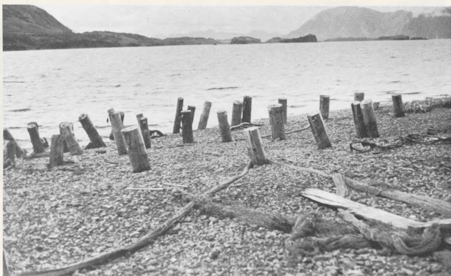
7. — Timber pile foundation at Kodiak Fisheries cannery site. Pronounced tilting of unbroken piling is indicative of lateral motion of the piling through 10–15 feet of beach gravel. Piling tops formerly level are now 7.8 feet lower at the seaward end of the cannery site than in the foreground owing to local settlement of the distal part of the beach culsp. Bent drift pins in the piling tops indicate that the cannery moved southward (away from the observer) off the piling.
