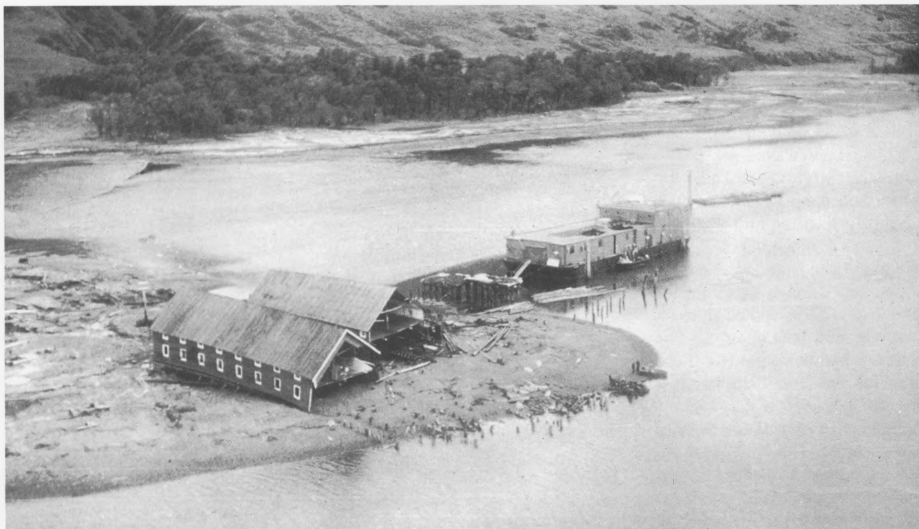
6.— The Kadiak Fisheries cannery site in Shearwater Bay along the north shore of Kiliuda Bay. Cannery buildings in the foreground were split during the earthquake and the seaward parts of the structures were later washed away by seismic sea waves. The former locations of the buildings and dock are outlined by timber pile foundations in the beach and water. The entire beach is now inundated at high tide as a result of about 4 feet of tectonic subsidence and 2-10 feet of surficial subsidence of the beach deposits. The barge behind the cusp is a floating cannery that replaces the destroyed facility on land. Location of cannery shown on figure 5.
