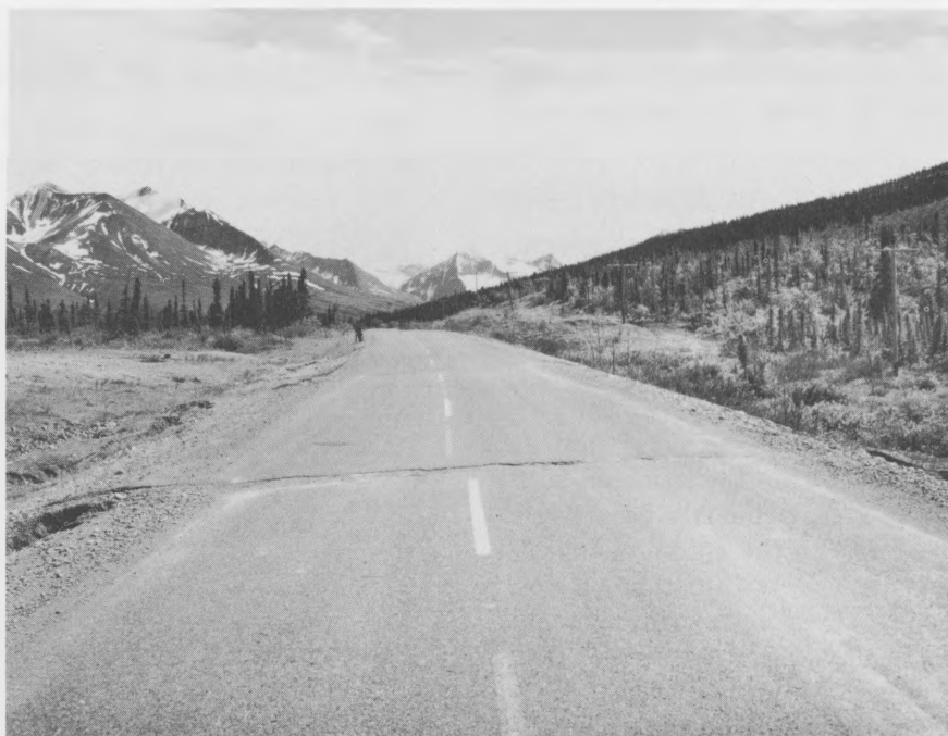
21.—View, to the southeast, showing the pavement surface of the Richardson Highway just south of the Little Tonsina River bridge at mile 65. Note the 8-inch horizontal offset of the centerline; vertical displacement is as much as 3 inches.
