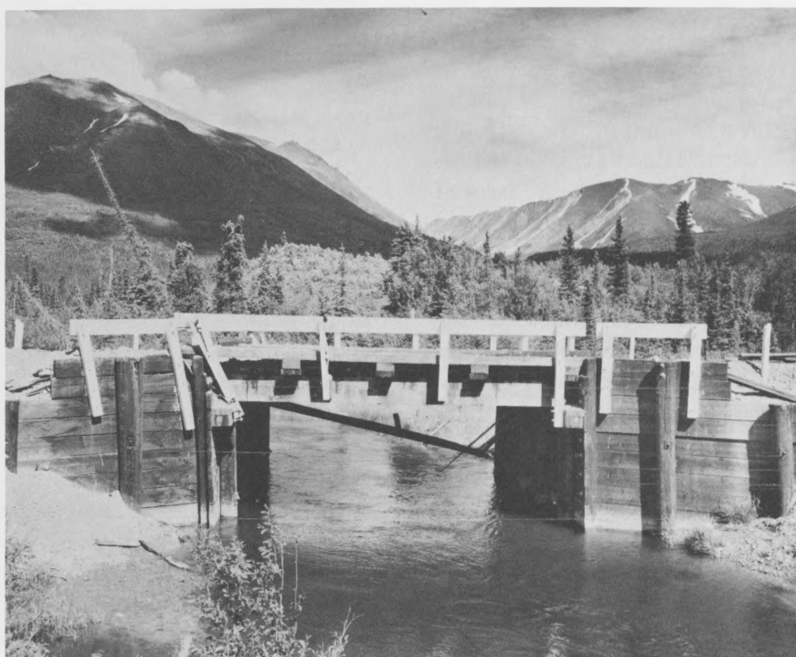
22.—Landslide movement on a hillside approximately two-tenths of a mile away caused the Little Tonsina River bridge to be shoved from the right to the left. Minor slumping occurred in road fill to the left of the bridge. Immediately after the earthquake the pavement was buckled more than 3 feet high at the left end of the bridge.
