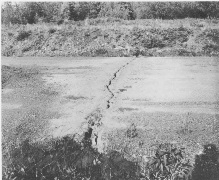
23.—Small crack across abandoned section of road on a low gravel terrace adjacent to Rock Creek at mile 86.1, Richardson Highway. Note the fine sand and silt along both sides of the crack.
