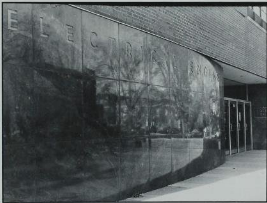
Coover Hall housed the electrical engineering facilities of the college. Engineering has been vital part to Iowa State and has earned an international reputation of excellence.
