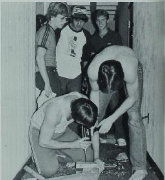
Above: The sound of hammers and drills are quite familiar on many dorm floors, especially during the first weeks
