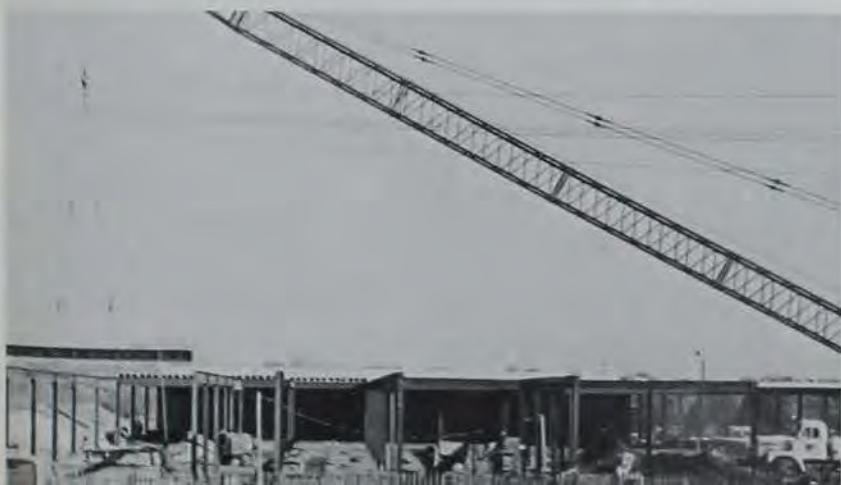
Seed Lab: In early phase of construction.
