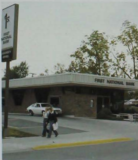
University Office Campus 2320 Lincolnway
