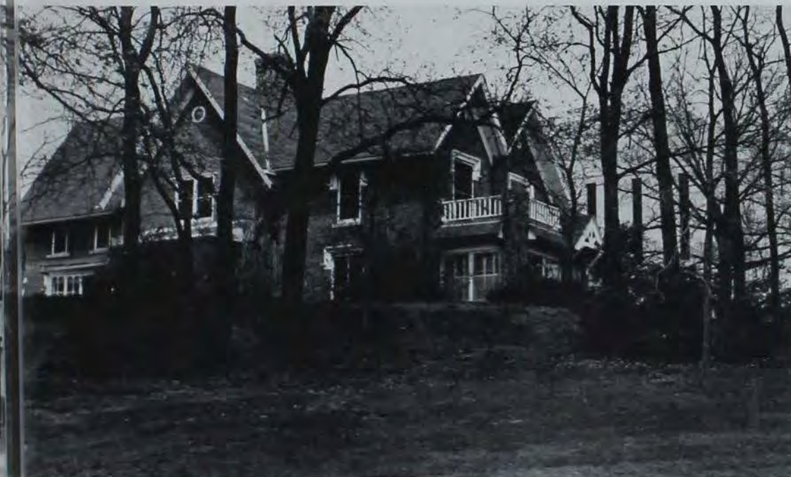
Music Hall had sat atop this hill on central campus since 1869. The building was razed last summer. Photos by John Riches
