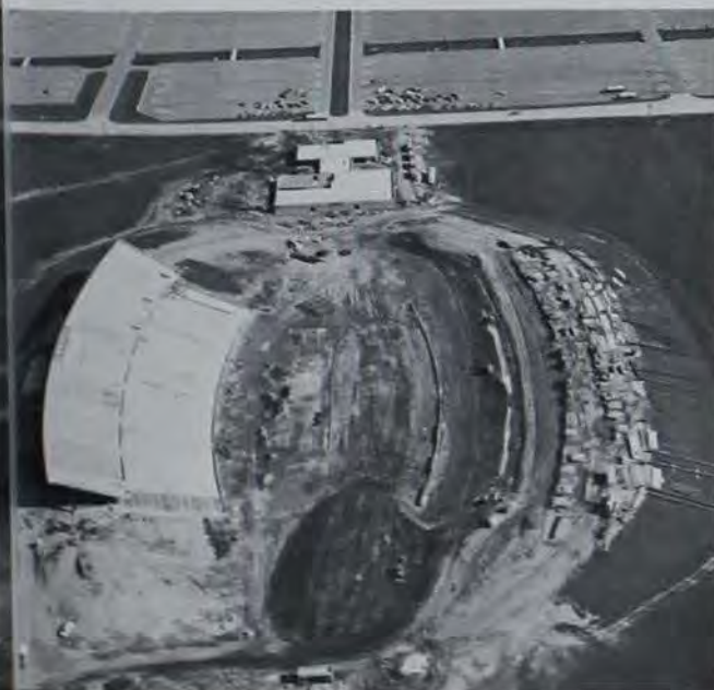
(Left), a look at the stadium in August 1974 after the east stands were torn down because of settling, and (right), nearing completion in December.
