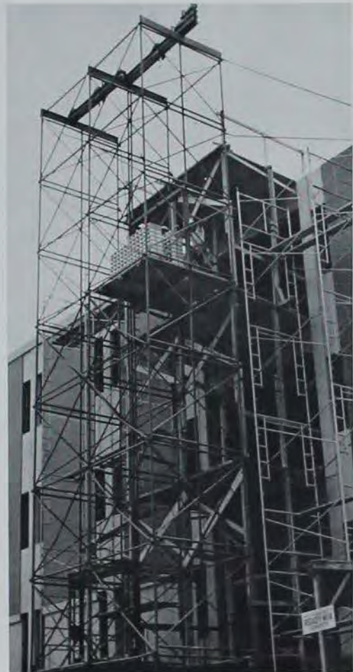
ANOTHER NEW BUILDING—animal science—takes shape as construction progresses on the campus.
