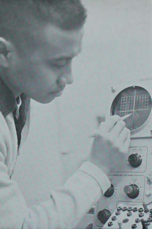
IN ELECTRONICS lab a vacuum tube curve tracer is all this student needs to evaluate quiescent operating conditions.
