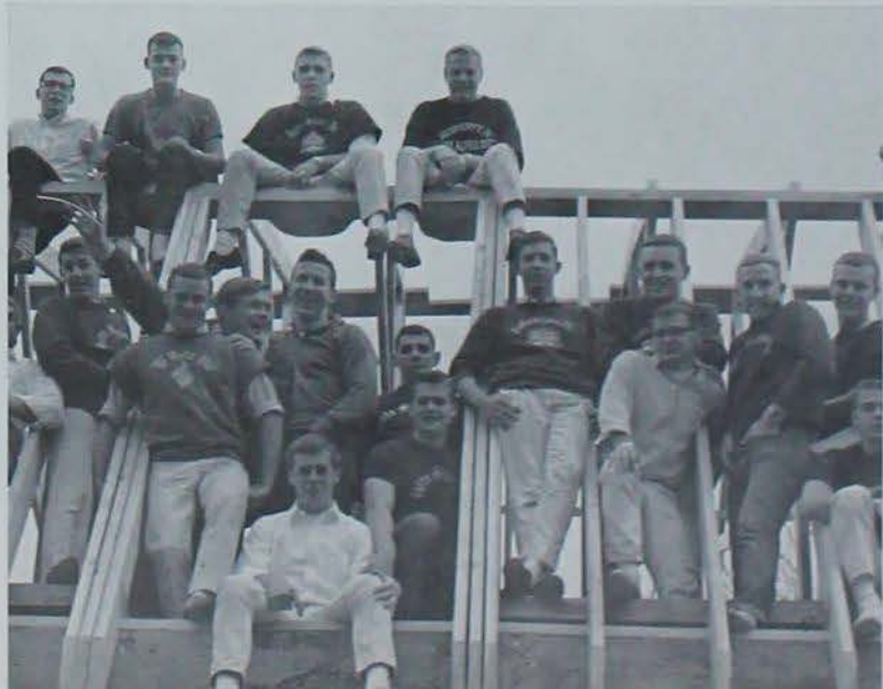
DELTA SIGS raise the room and build their new addition.
