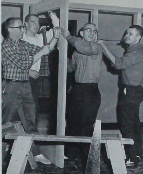
A GLASS WALL is installed as part of the remodeling work on the Cessna House den. Dens in Friley-Hughes Hall are being remodeled at the rate of two per year.
