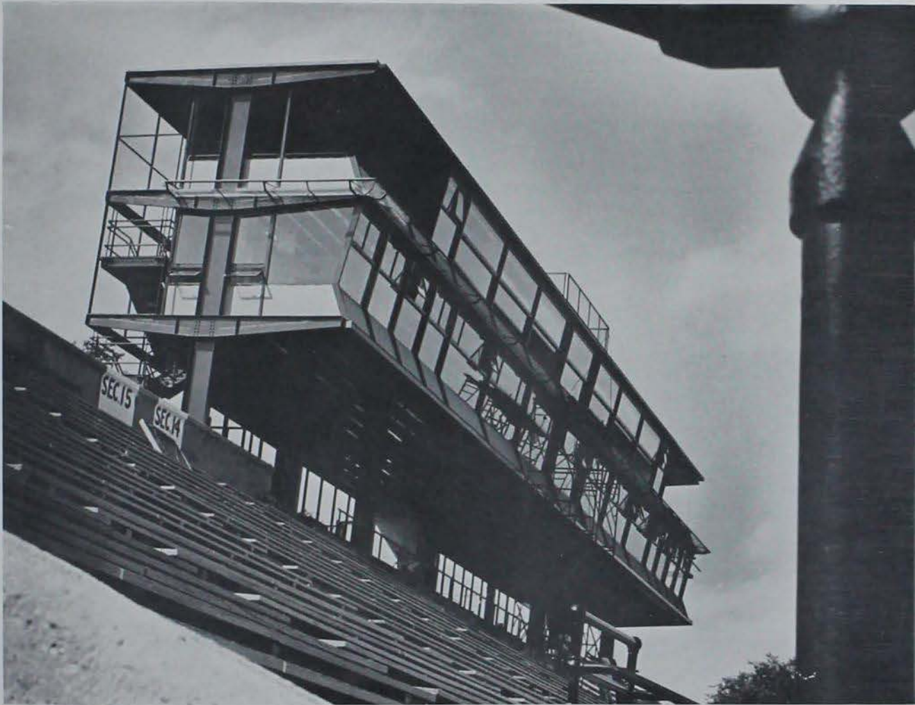
TAKING ITS PLACE in the Clyde Williams Field Stadium, the double-decker press box, complete with elevator, accommodates about fifty newsmen, announcers, and technicians.
