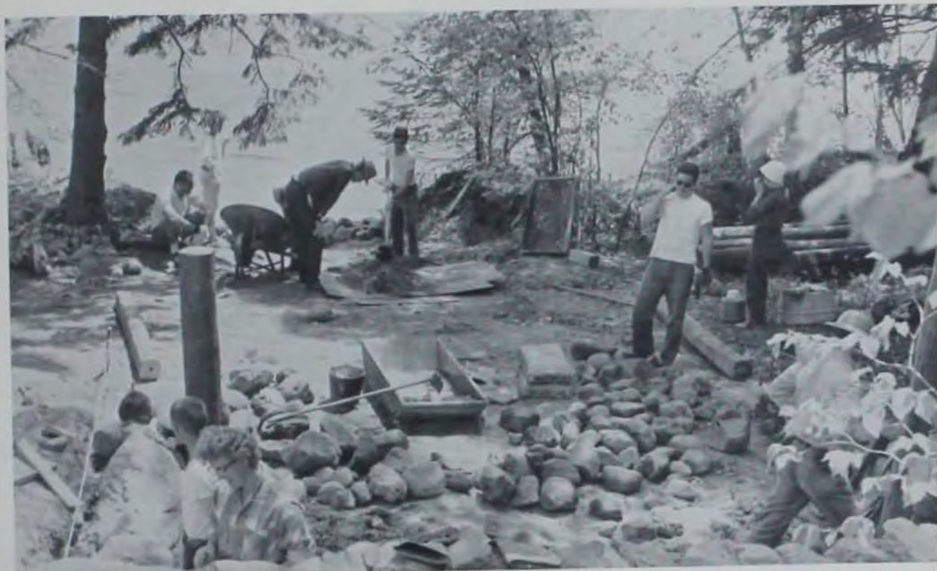
CONSTRUCTION PROJECTS are a part of church-sponsored summer work programs, which also include training in youth counseling, migrant ministry, settlement and social work.
