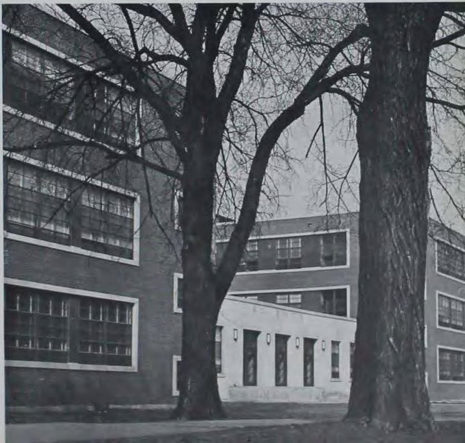
The new Science Building peacefully awaits the swarms of students early in spring quarter.
