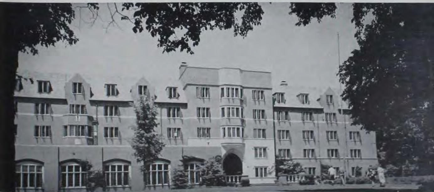
Friley-Hughes Hall, sprawling men's dormitory on the west edge of the campus, was built in 1939. Additions to the building in 1942, 1950 and 1954 brought total investment to $2,587,665.
