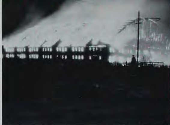
A spectacular blaze in 1922 left the college Armory in skeleton form. Destruction was $260,000. A second building, similar in design, was constructed the following year on the same spot.
