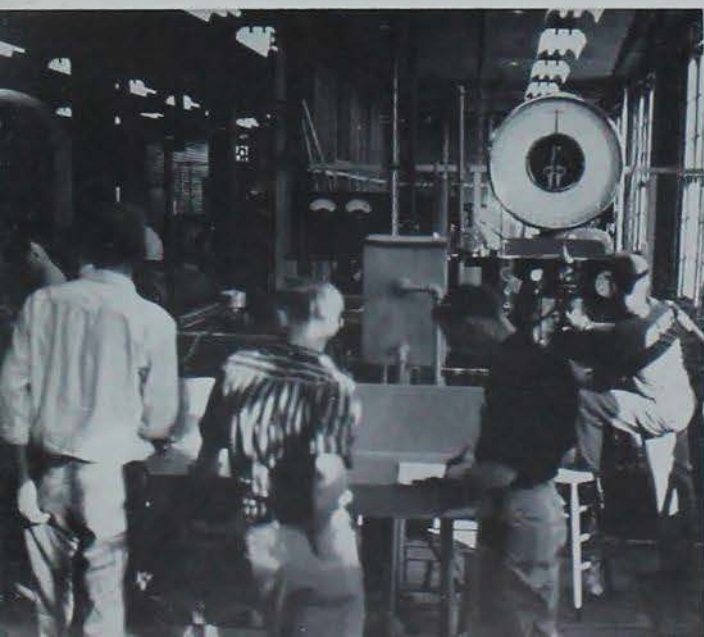
Scientific and mathematical principles are applied to the field of mechanics in the mechanical engineering department. Here seniors test the performance of an internal combustion engine.
