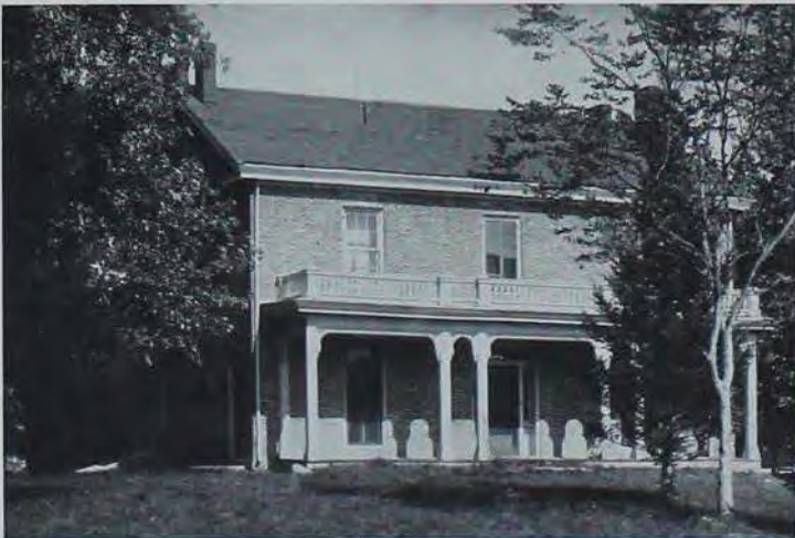
In 1861 the Farm House, first campus building, was erected. For many years the residence of superintendents of the Model Farm, the house is presently occupied by the Dean of Agriculture.
