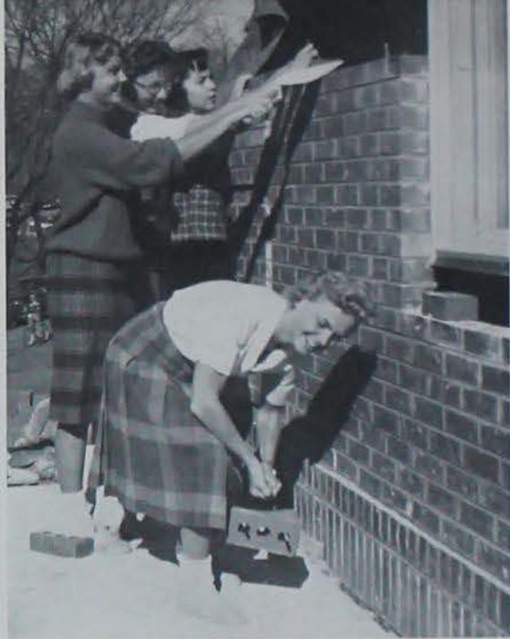
FOUR ALPHA GAM's try laying bricks as they help in the building of their new addition, scheduled for completion in January.
