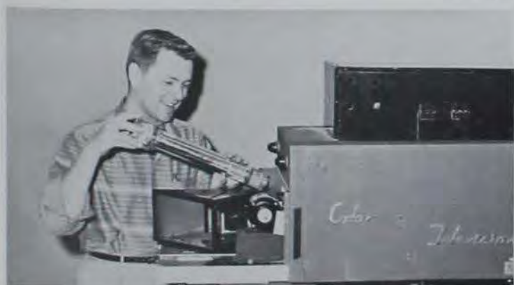
ADJUSTING OPTICS on a color television camera is Delbert Whitmer, research technician at the Engineering Experiment Station. The station is trying to perfect a simplified system for transmitting color television signals which the university developed.
