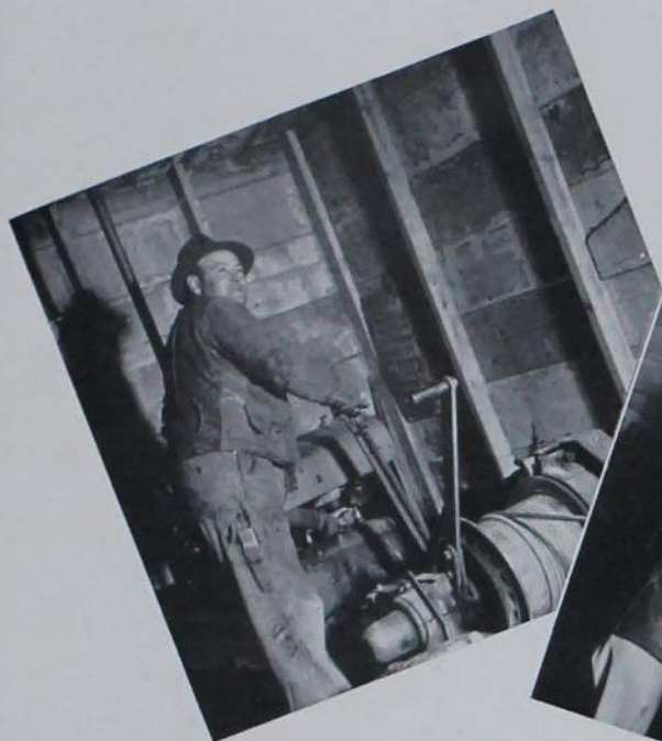
Hoisting materials for the new addition
