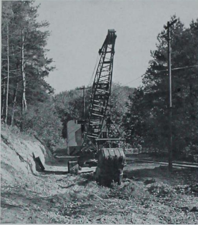
This shovel chewed out a new drive below the Union.
